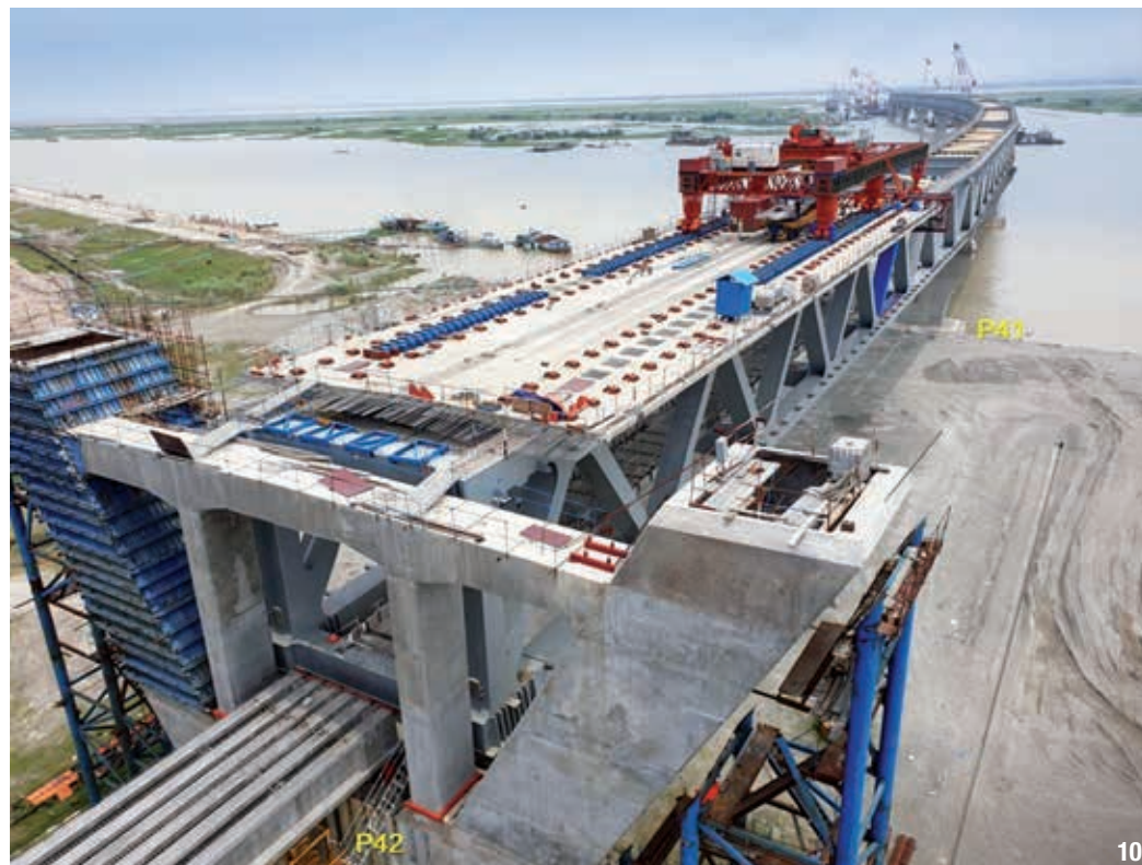
10- Assembly of first deck panel launching gantry. 11- View of approach viaducts from Janjira side.
