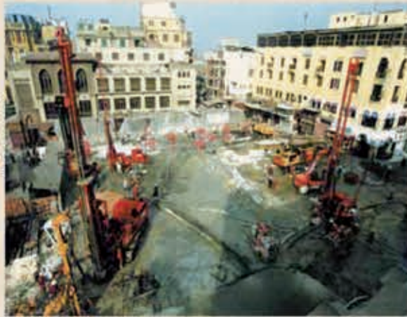
Photo 7 L'hydrofraise à Port Said en action The hydro-cutter in action at Port Said
