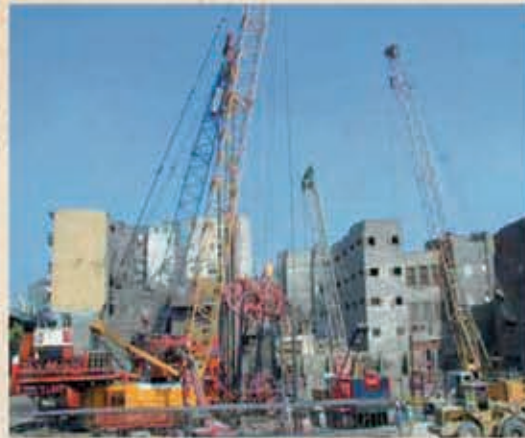
Photo 7 L'hydrofraise à Port Said en action The hydro-cutter in action at Port Said
