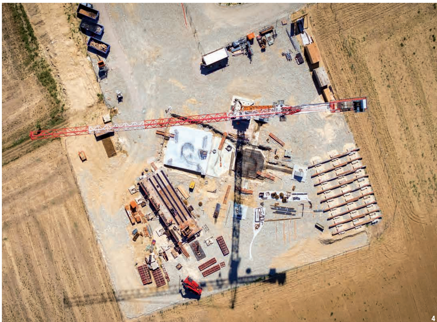
4- General view of the site and the crane.
