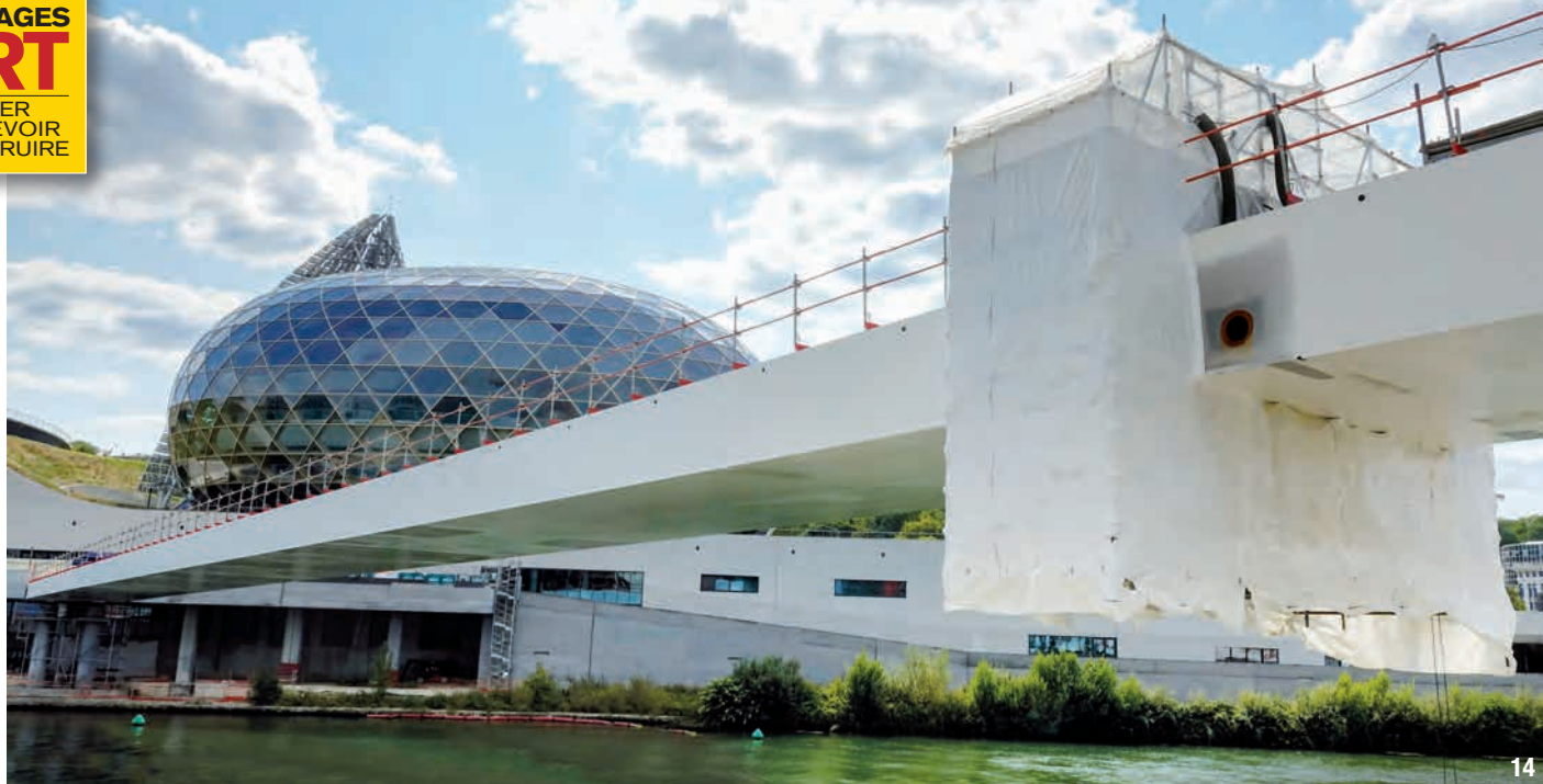
© VICTOR BUYCK STEEL CONSTRUCTION 14
