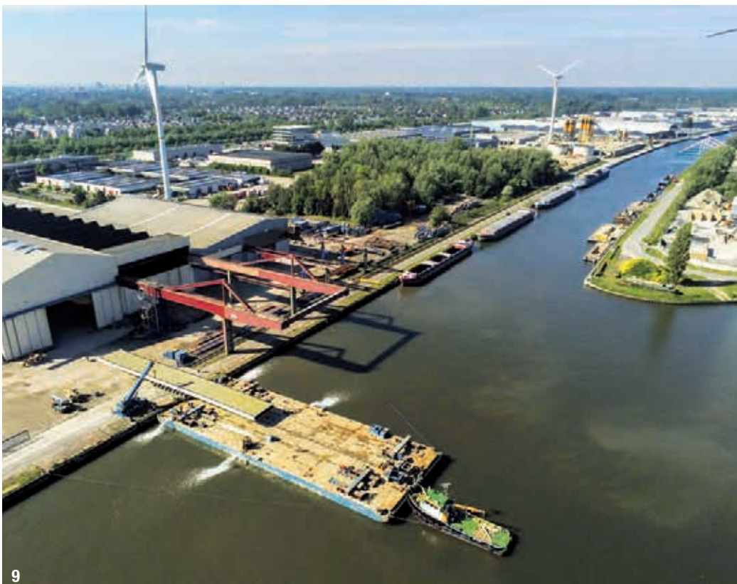
9 © VICTOR BUYCK STEEL CONSTRUCTION
