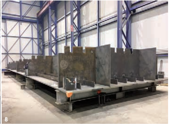
8 © VICTOR BUYCK STEEL CONSTRUCTION
