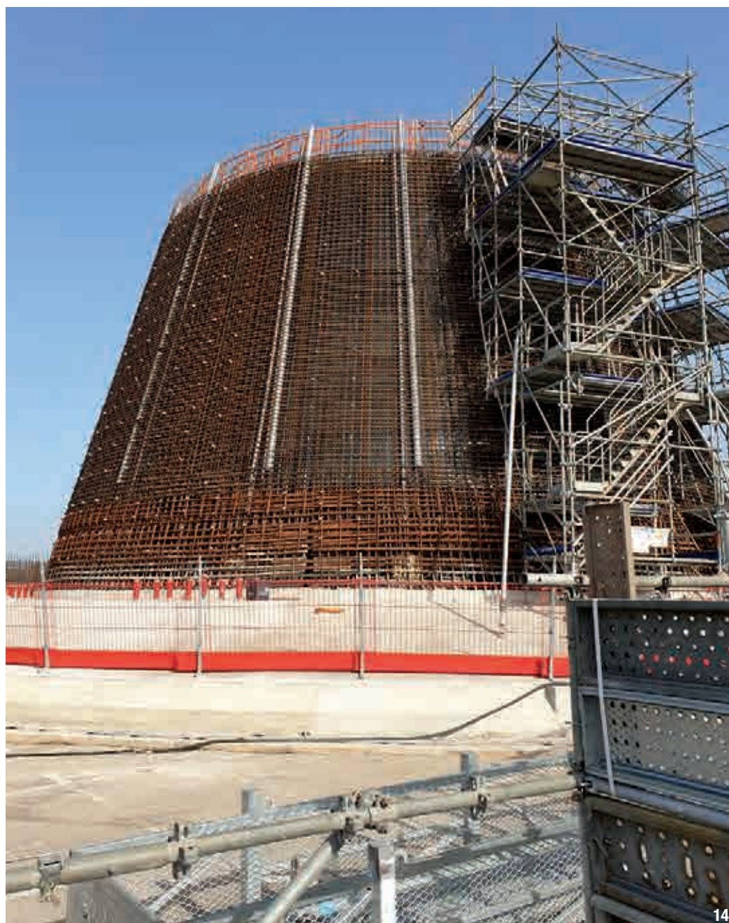
13- Rebars of the bottom lifting pad. 14- Rebars of concrete lift 1 for a shear wall.
