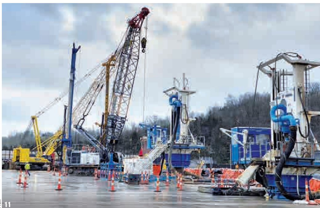
10- View of the project during the works phase. 11- Reverse circulation drilling (RCD) rig.
