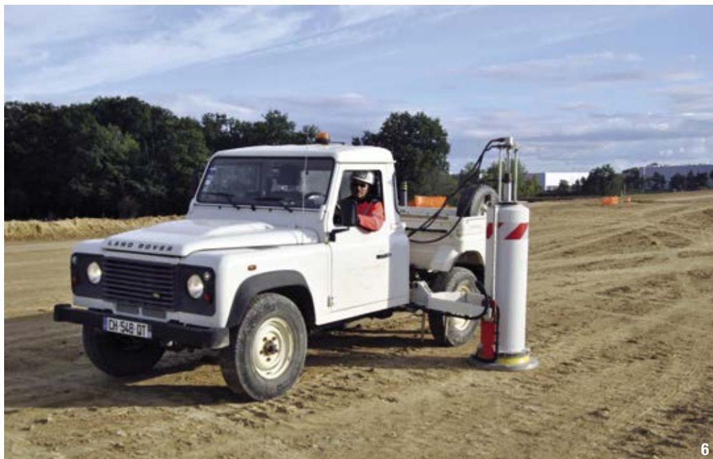
© VINCI CONSTRUCTION TERRASSEMENT
