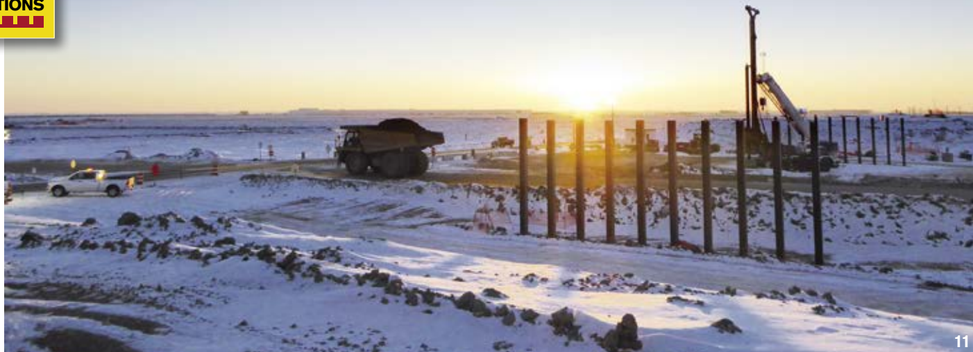
© VINCI CONSTRUCTION TERRASSEMENT
