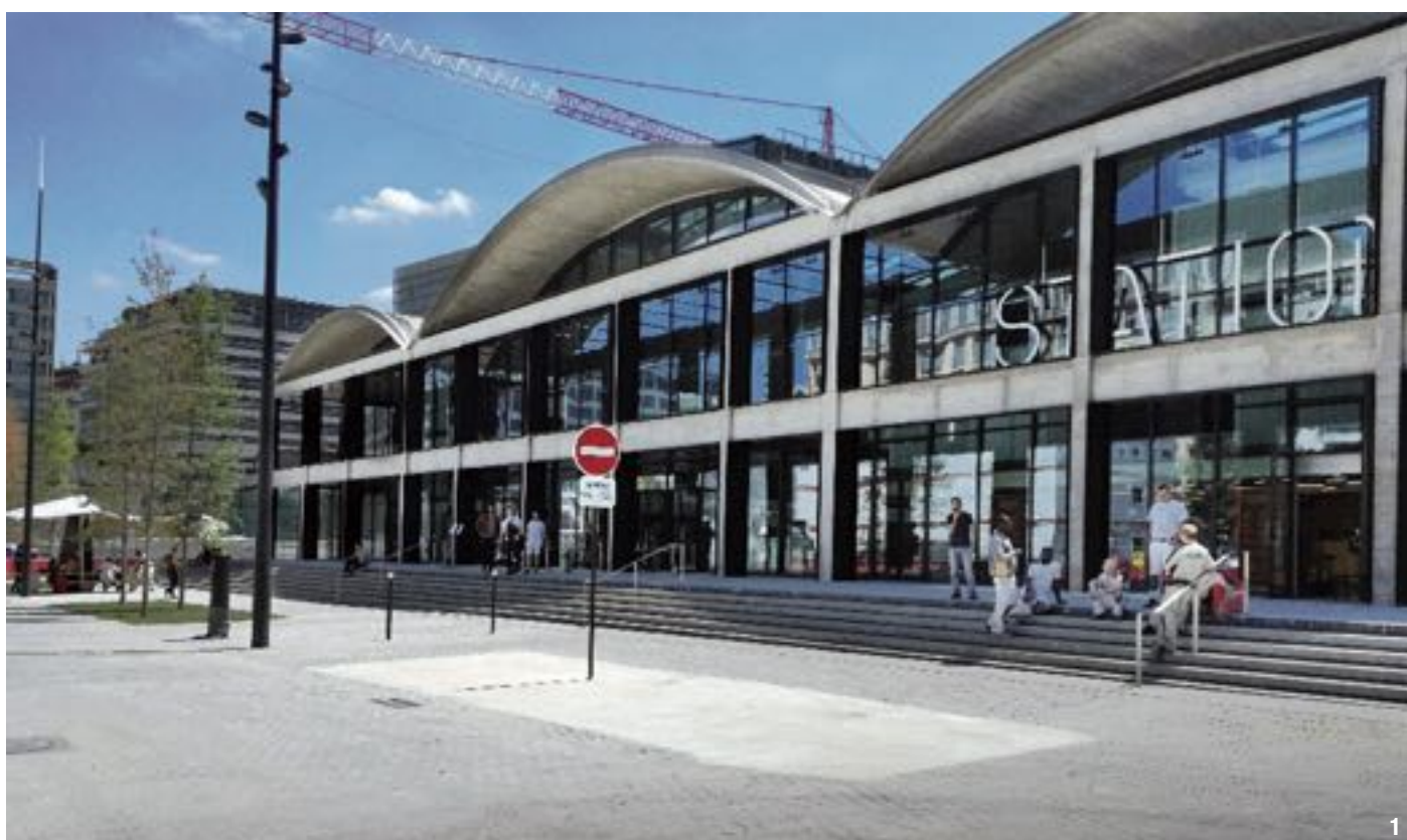
© PHOTO THÈQUE ARTELIA 1
