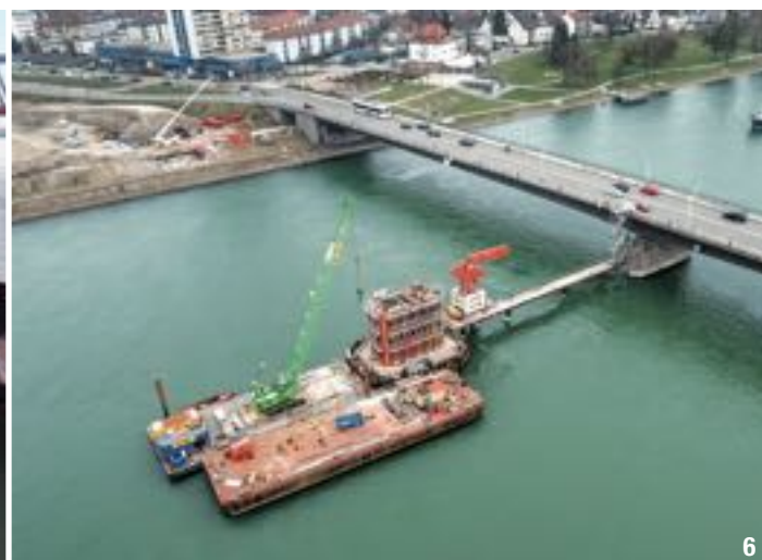
FIGURE 5 © ARCADIS - FIGURE 6 © BOUYGUES
