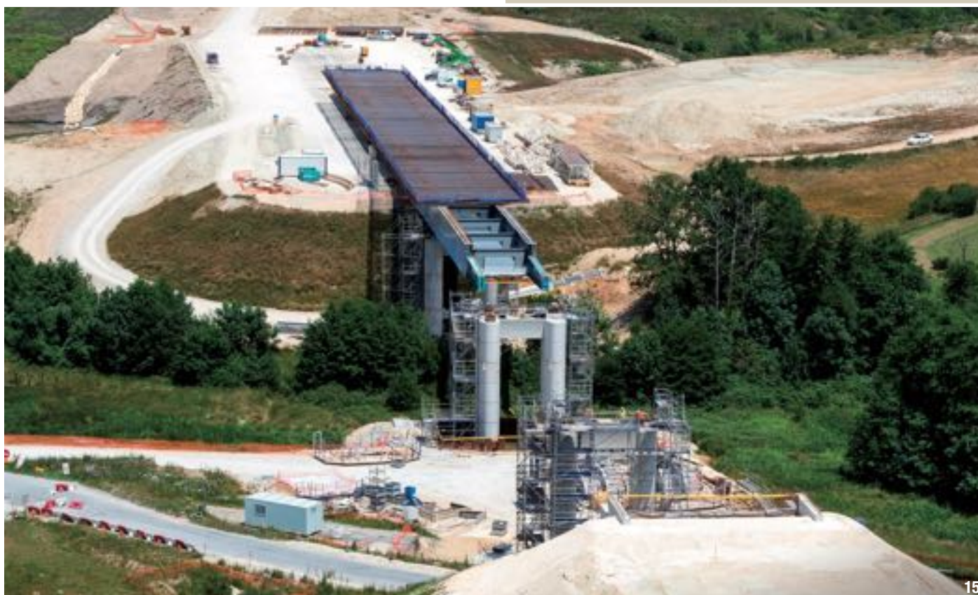
15- Launching the deck of the Palais viaduct (VIA 2507).
