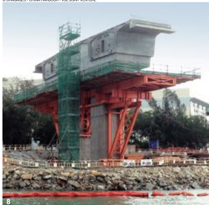
© DRAGAGES - CHINA HARBOUR - VSL JOINT VENTURE
