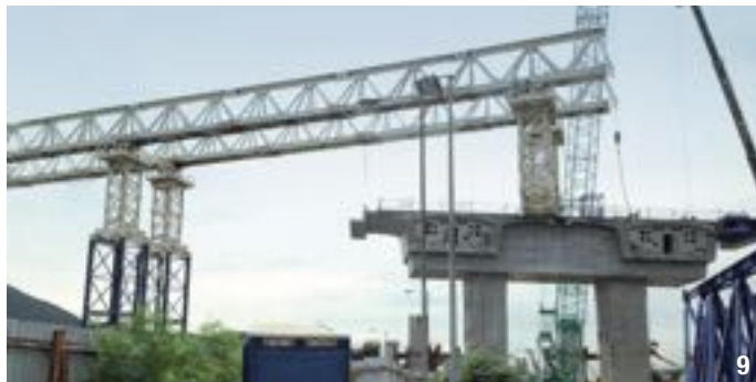
9 © DRAGAGES - CHINA HARBOUR - VSL JOINT VENTURE
