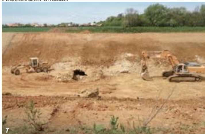
© VINCI CONSTRUCTION TERRASSEMENT
