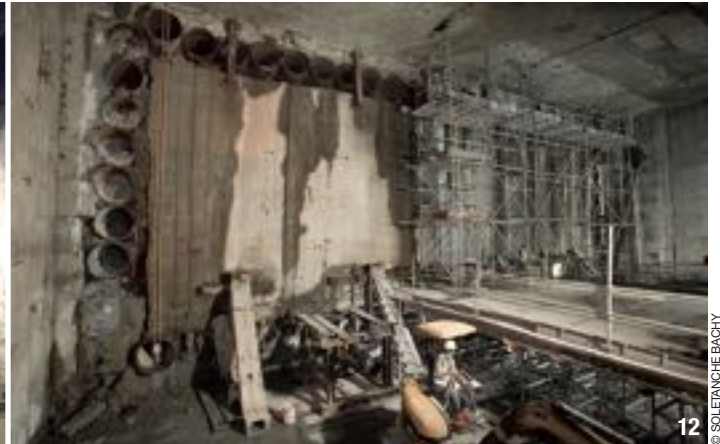
11- Setting up and welding - Beach Road rail tunnel. 12- Temporary propping to support diaphragm wall. 13- Pipe jacking and mining - South Wing. 14- The "Gun" for the Ø600 pipes. 15- Drilling in the soil nails using the Springsol. 16- The Springsol tool, unfolded.
