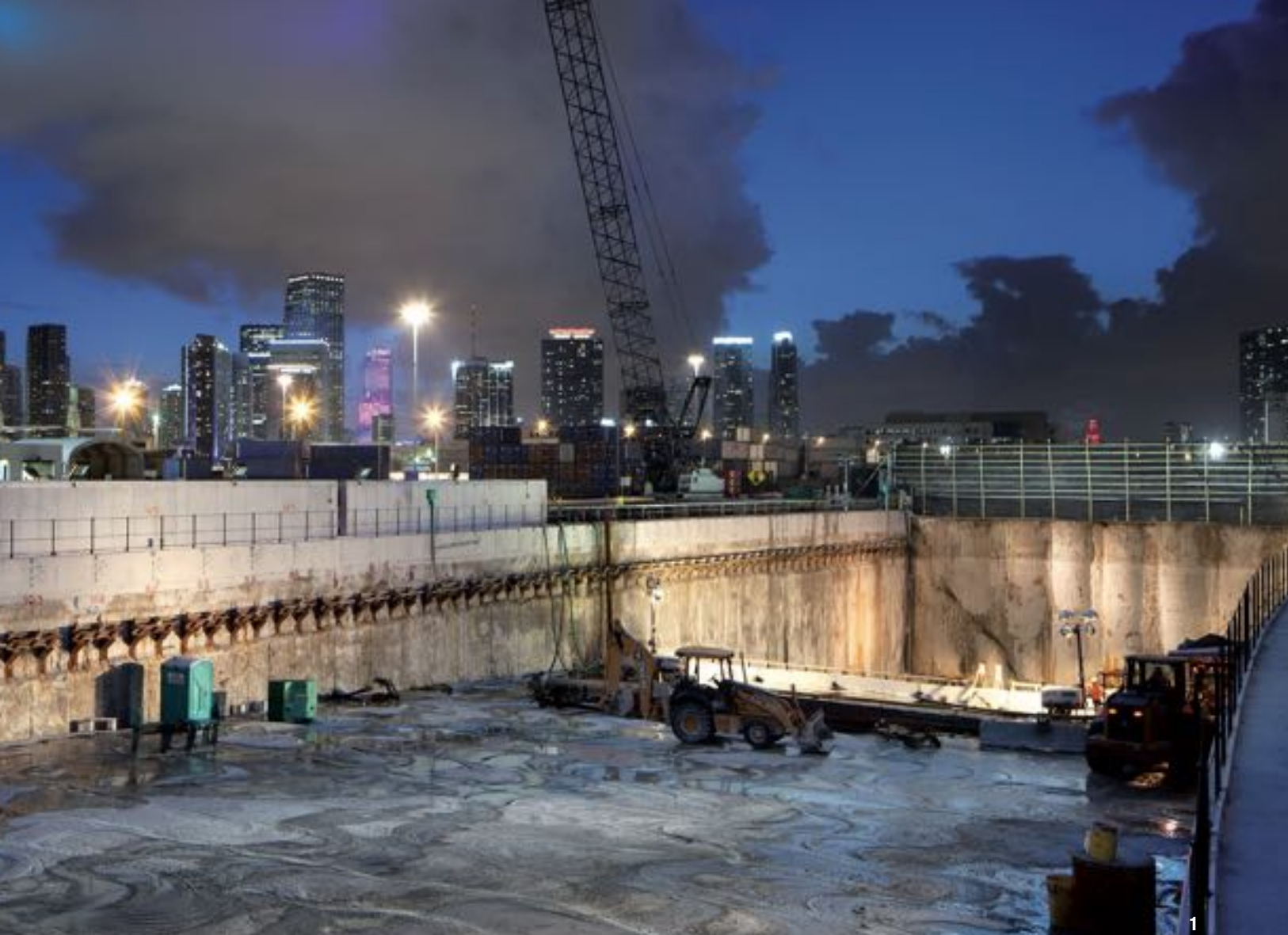
1 © MALCOLM DRILLING COMPANY
