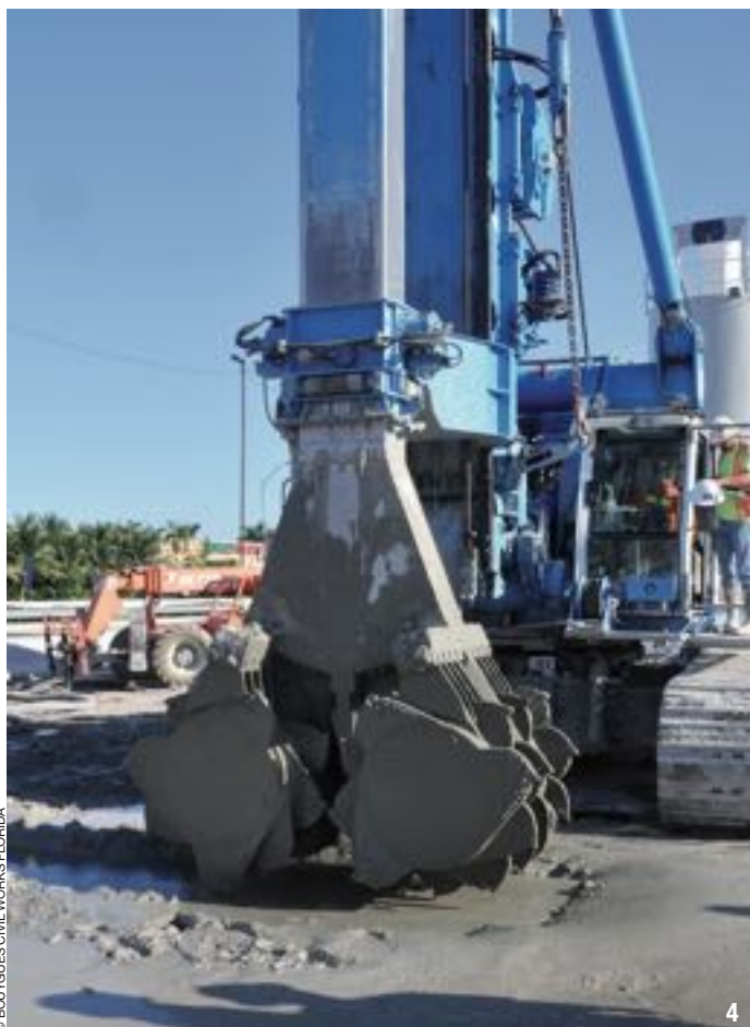
© BOUYGUES CIVIL WORKS FLORIDA
