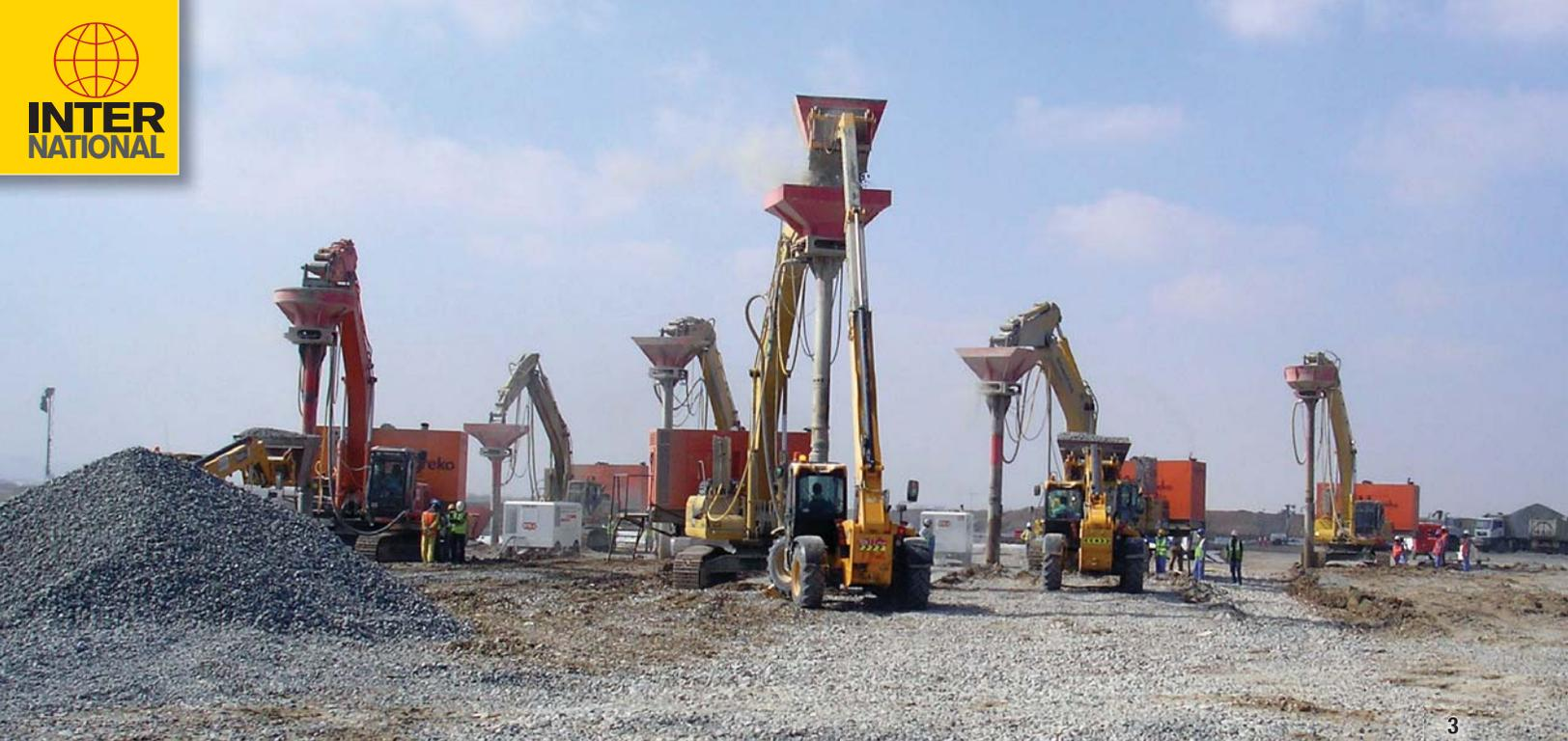
and further CPTUs (one per 900 square metres) were undertaken. The principal method of post treatment testing is by CPTU, which are being undertaken at the centroid of triangles formed by the stone columns.
