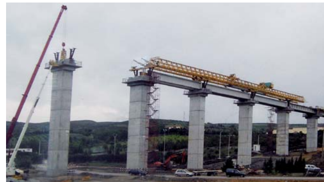
10- Viaduct at PK6 – Launching girder.
