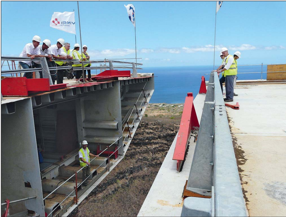
Photo 22 Derniers mètres avant clavage Final metres before keying
