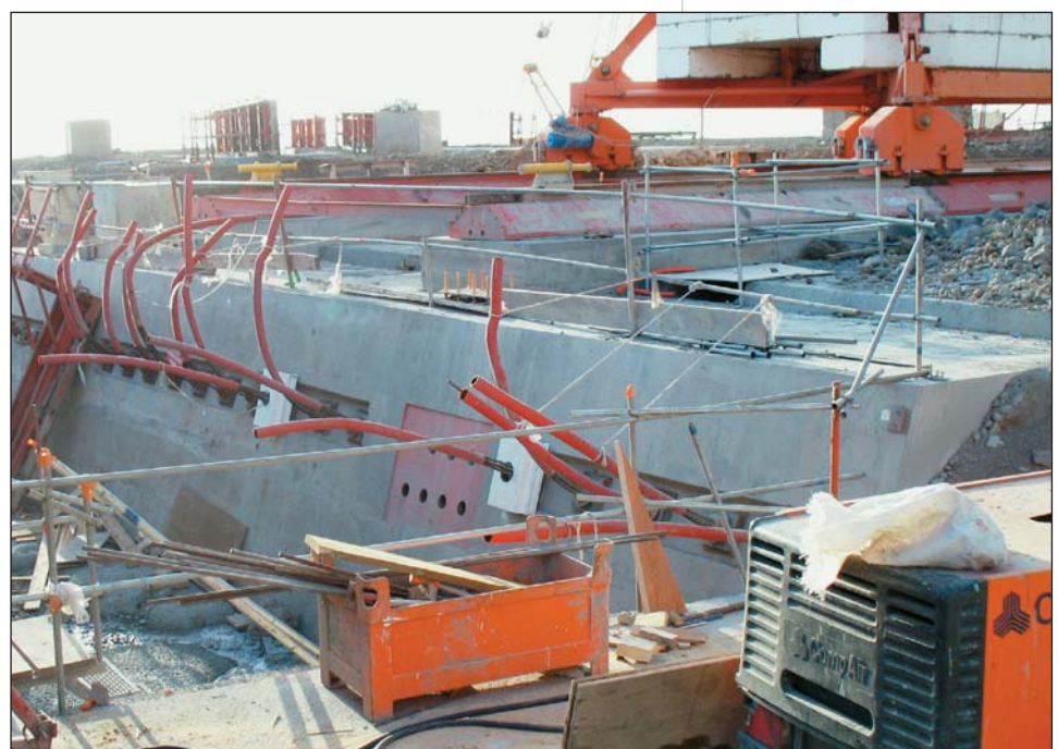
Photo 7 Massif de stabilisation terminé Completed stabilisation foundation block
