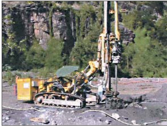
Photo 7 Jet grouting Jet grouting
