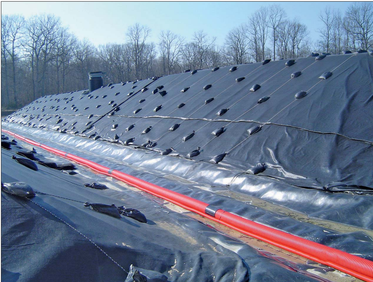
Photo 10 Protection et lestage Protection and ballasting
