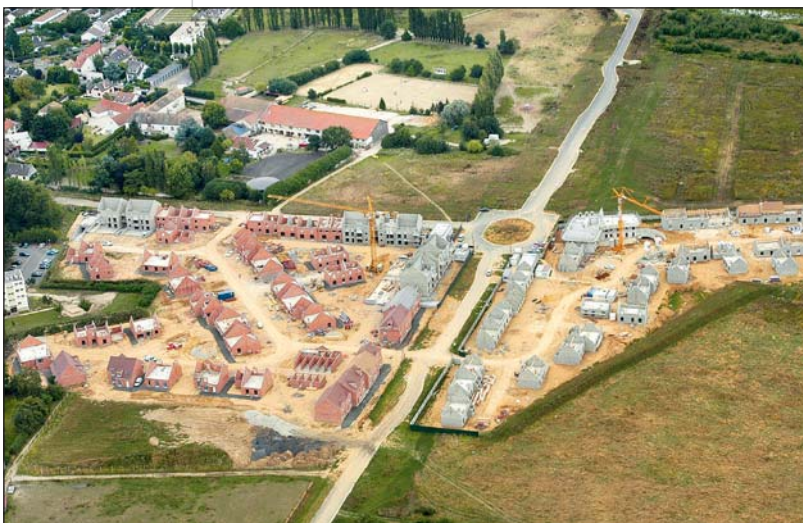
Photo 2 Lotissement en construction Housing estate under construction
