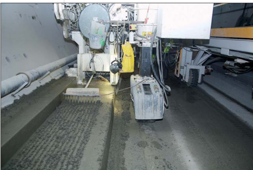
Photo 9 Semelle quai haut Footing of high quay
