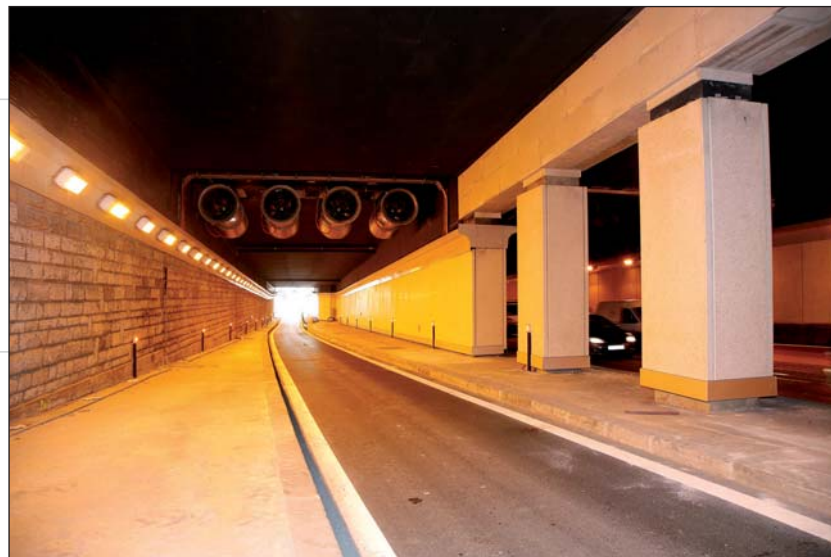
Photo 8 Habillages architecturaux du tunnel Architectural facings of the tunnel
