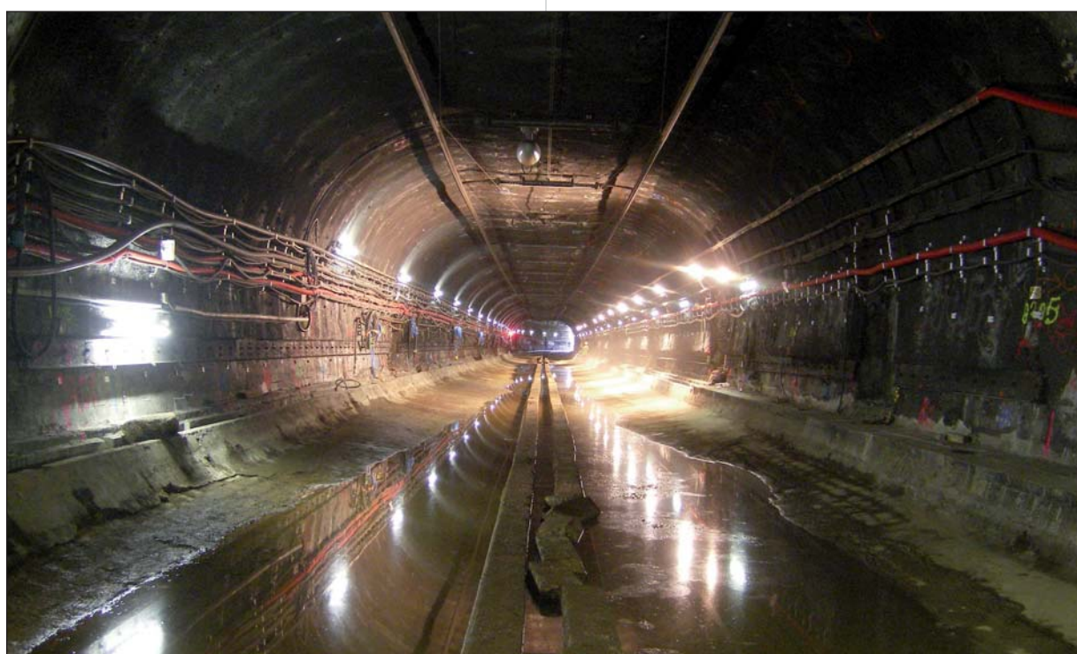
Photo 2 Vue du tunnel View of the tunnel
