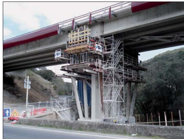
Photo 2 Palée provisoire Temporary bent
