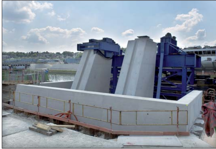
Photo 3 La pile P1 Pier P1
