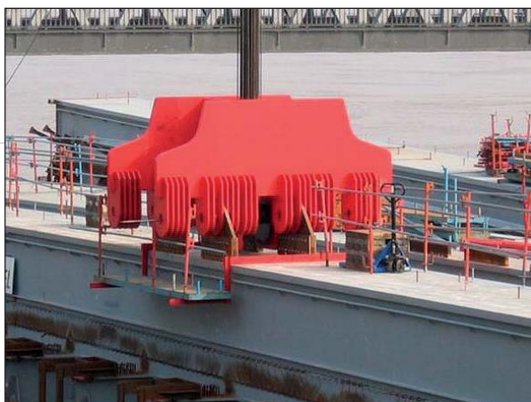
Photo 16 Palonnier de levage multipositions Multi-position lifting beam
