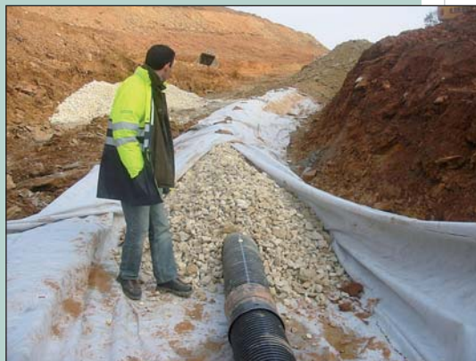
Photo 9 Tranchée drainante Drainage trench
