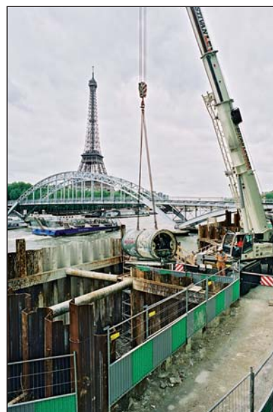
Photo 7 Descente du tunnelier TBM lowering
