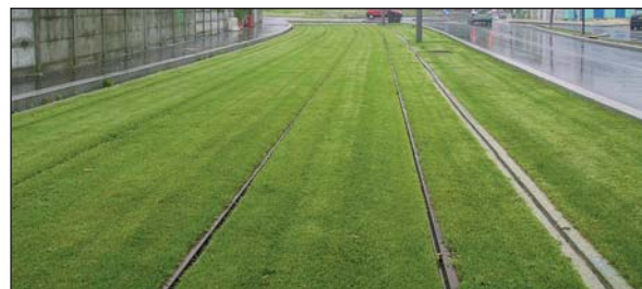
Photo 6 Voie engazonnée - Solution traditionnelle Track planted with grass - Traditional technique
