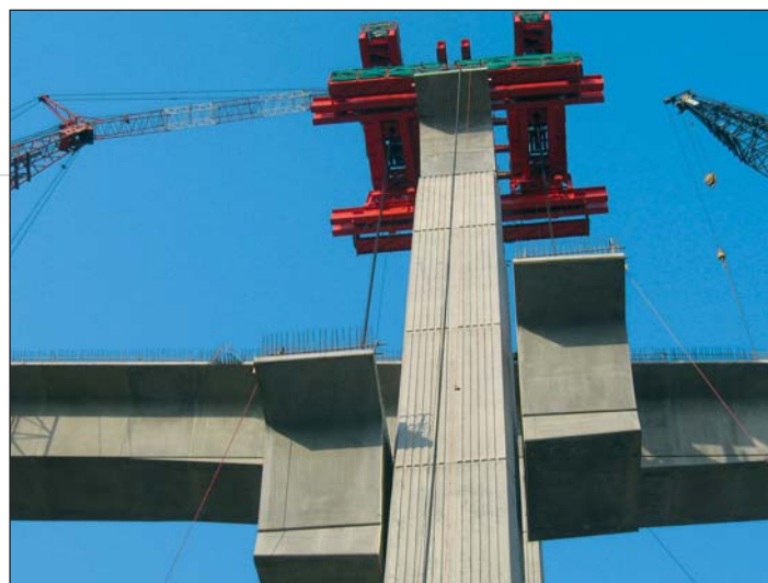
Photo 10 Chèvre pendant levage Tripod derrick during hoisting
