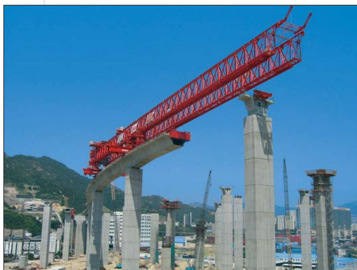
Photo 8 Poutre en configuration de lancement maximum Girder in maximum launching configuration
