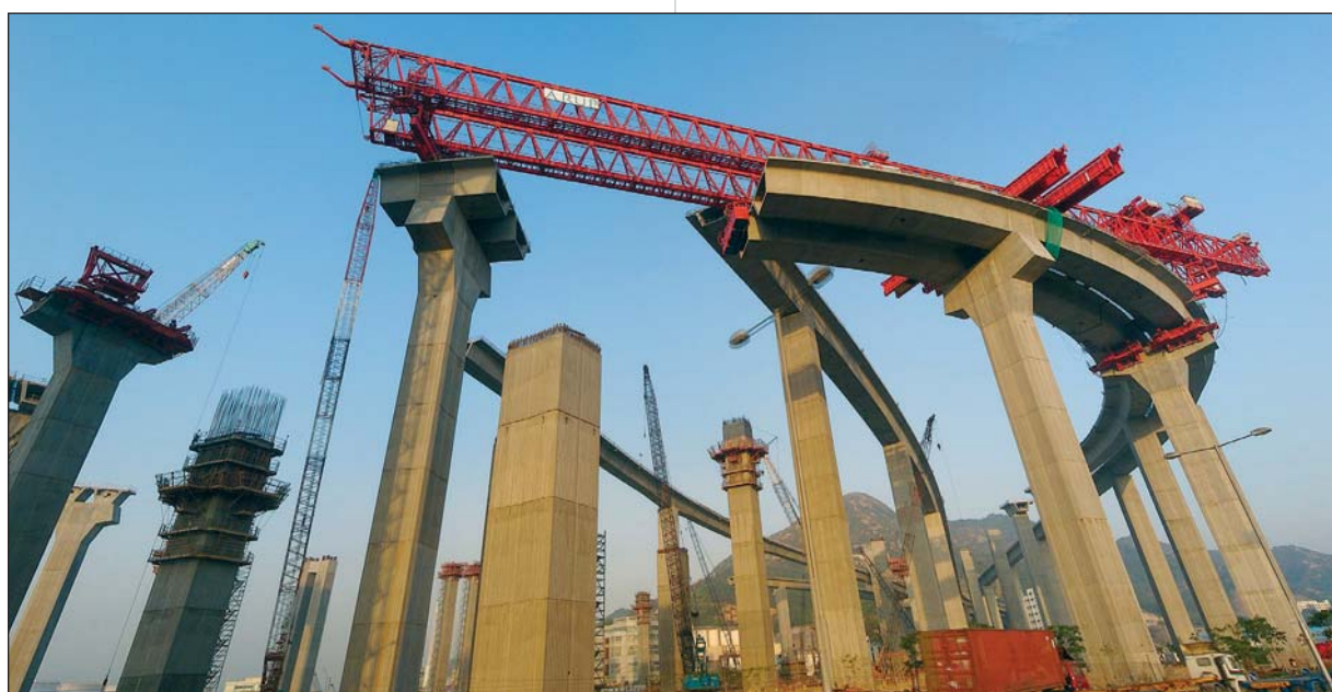
Photo 12 Vue de la pose en courbe View of placing in curve
