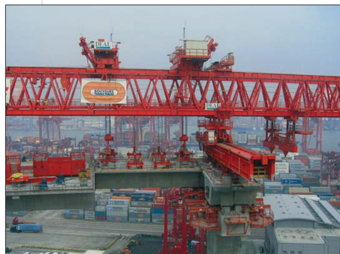
Photo 8 Poutre en configuration de lancement maximum Girder in maximum launching configuration
