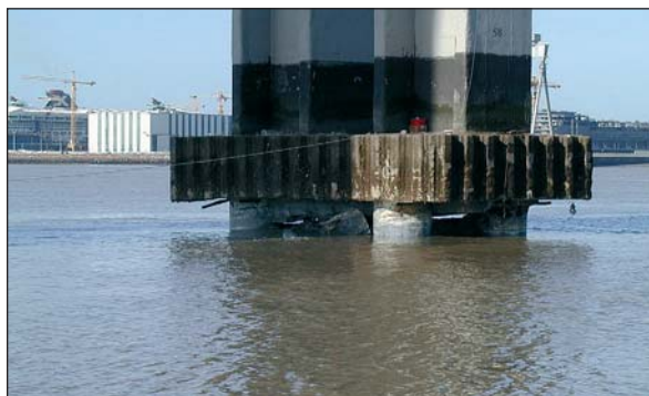
Photo 10 Semelle béton Concrete foundation slab
