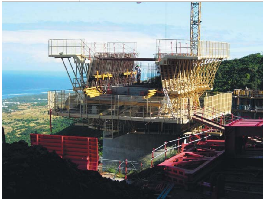
Photo 7 Coffrage du VSP Formwork for segment on pier
