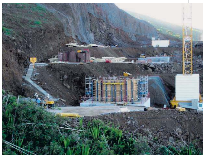
Photo 5 Coffrage pile P3 Formwork for pier P3
