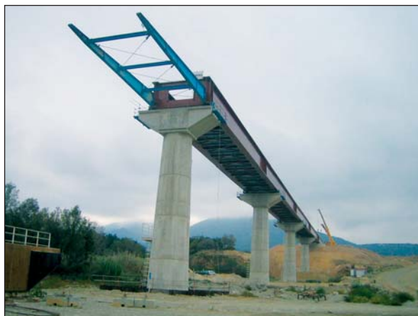
Photo 14 VIA 15.65 – Fin de la 1 re phase de lancement (septembre 2006) VIA 15.65 – End of the first stage of launching (September 2006)
