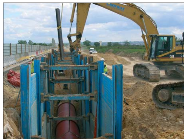
Photo 5 Pose en tranchée blindée Laying in shielded trench
