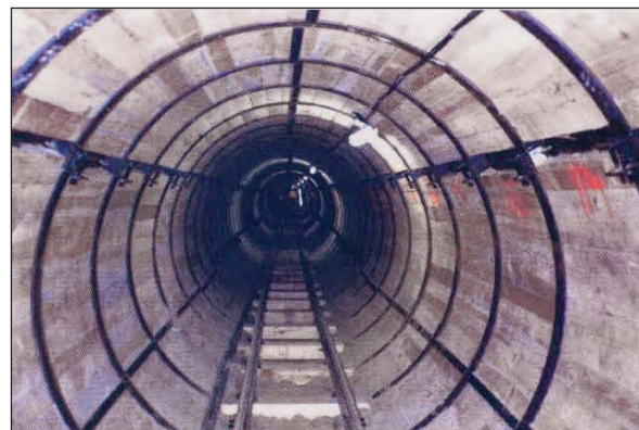
Photo 3 L'aspect du tunnel prérevêtu The appearance of the pre-lined tunnel
