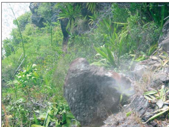
Photo 2 Purge de blocs Removing rock blocks
