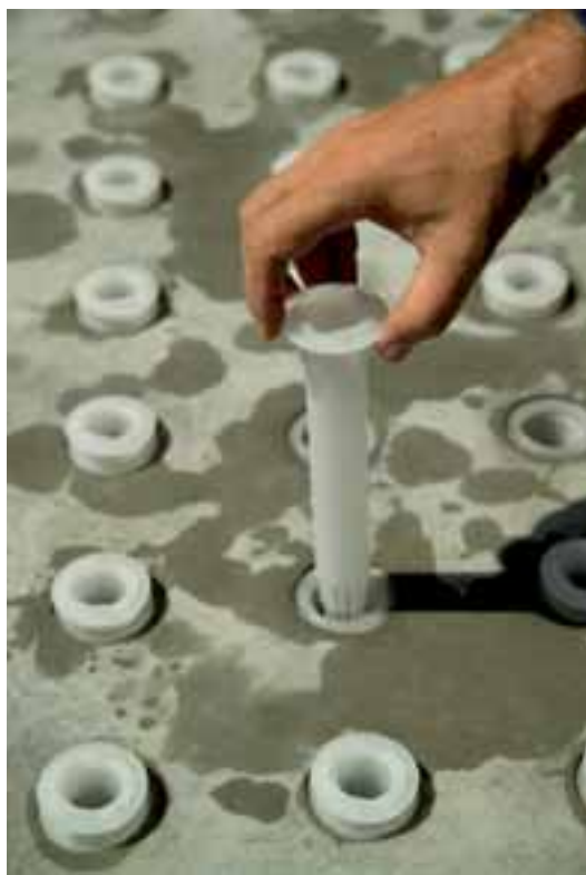
Installation de crépines Installing filter screens
