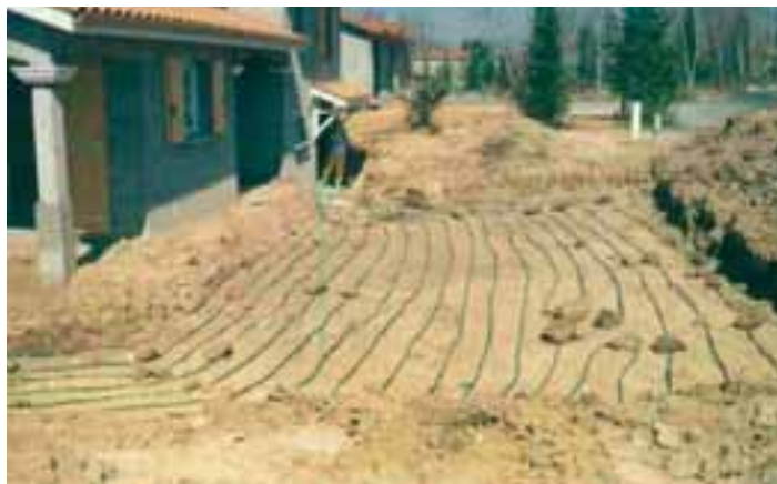
Installation géothermique en cours Geothermal heating installation work in progress
