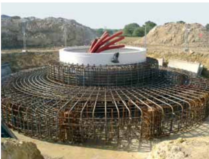
Photo 6 Massif béton armé Reinforced concrete foundation
