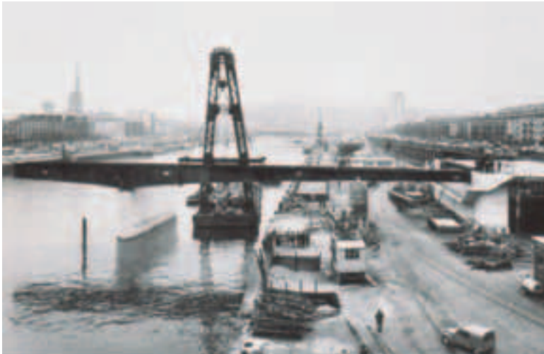
Photo 18 Exemple de bigue fluviale Example of heavy river derrick taken from BT8
