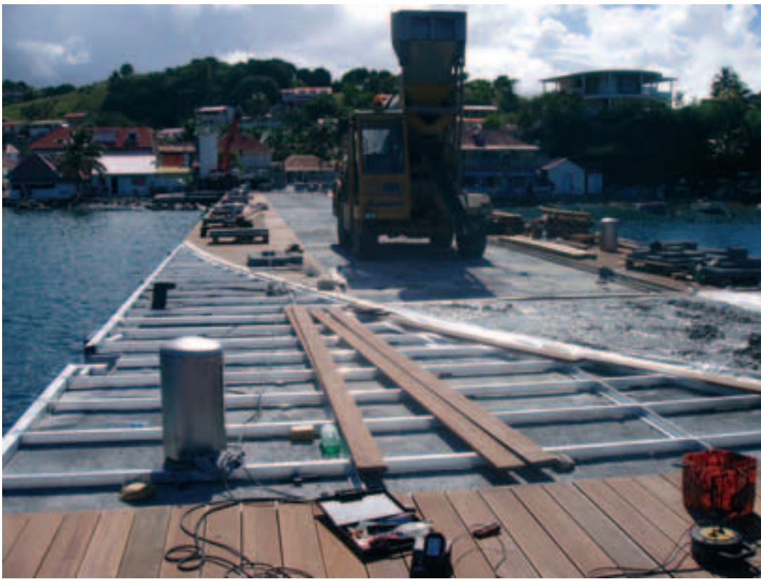
Photo 5 Construction du deck Construction of the deck
