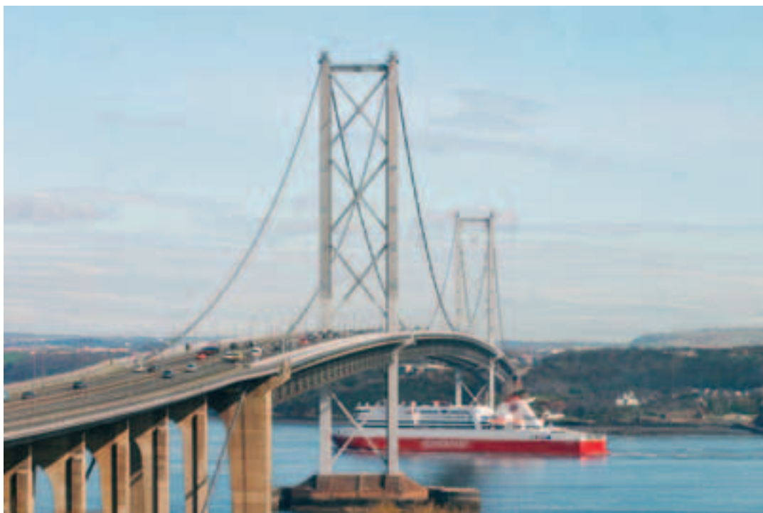
Forth road bridge Forth Road Bridge
