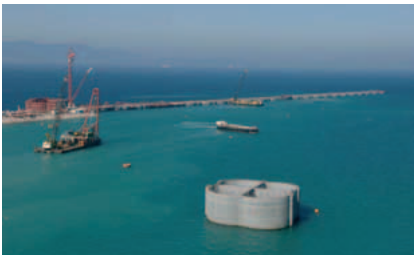
Photo 13 Remorquage du caisson Towing the caisson
