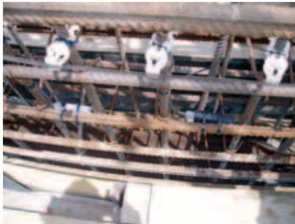
Photo 5 Rubans de la protection cathodique Cathodic protection tapes
