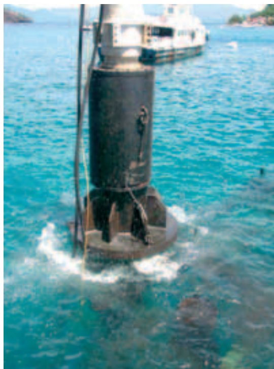
Photo 3 Fonçage au marteau hydraulique Pile driving by hydraulic hammer
