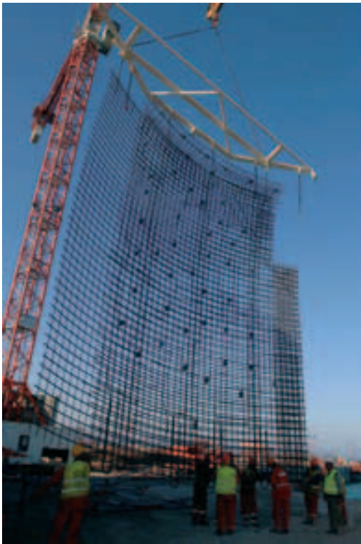
Photo 15 Levage cage d'armatures Hoisting the concrete reinforcing cages
