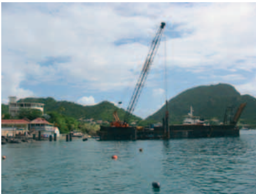
Photo 3 Fonçage au marteau hydraulique Pile driving by hydraulic hammer
