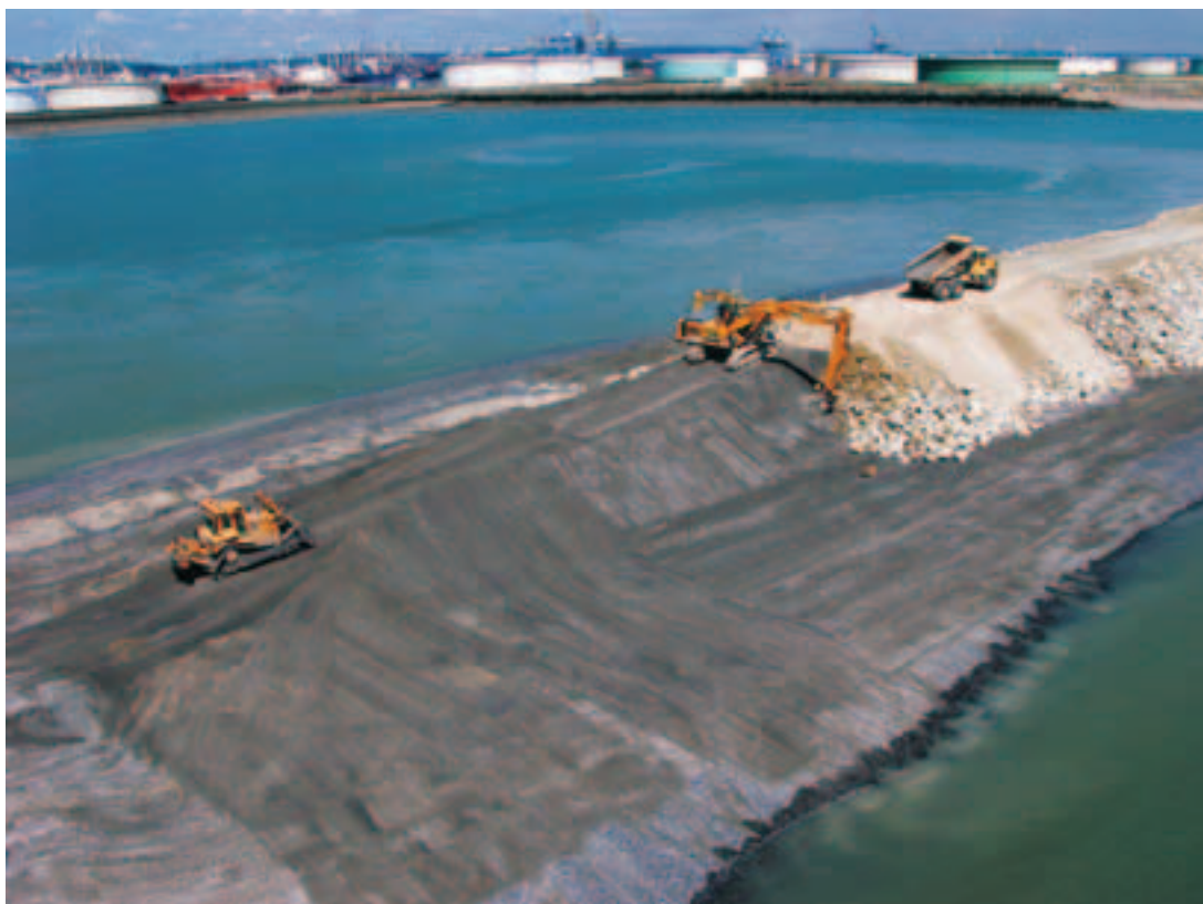
Construction of the outer breakwater of Port 2000
