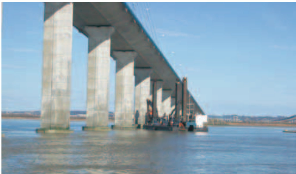
Photo 2 Protection des piles Protection of the piers
