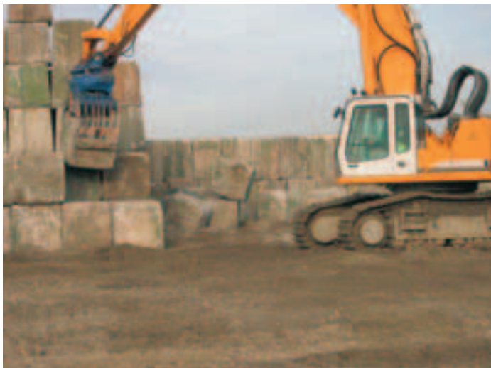
Photo 10 Stockage de blocs cubiques Storage of cubic blocks
