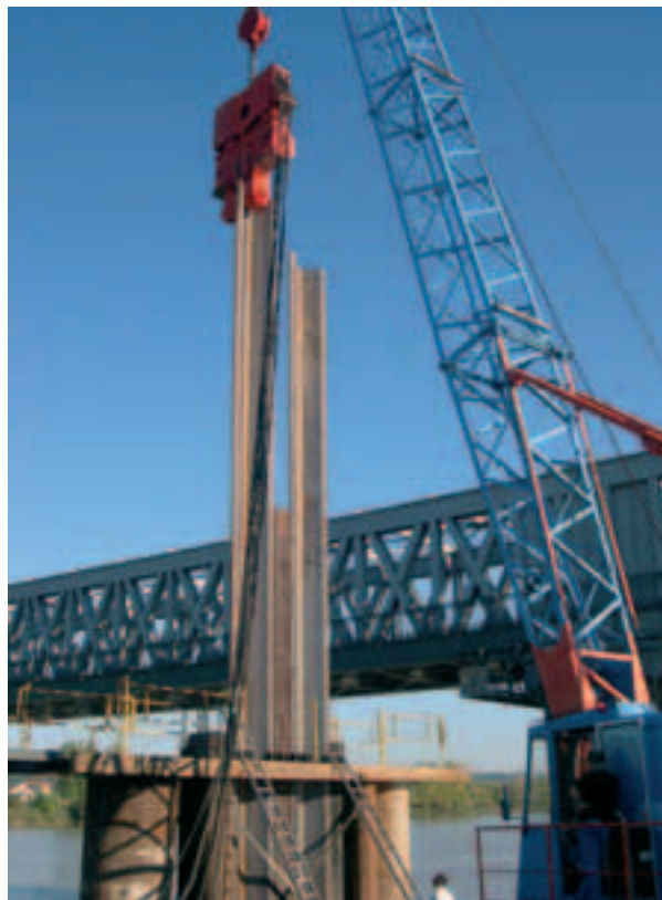
Photo 1 Essai de battage en rivière Pile driving test in the river
