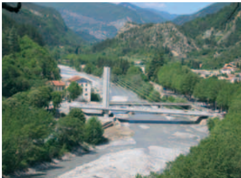
Photo 17 Vue de l'ouvrage terminé... General view of the completed structure
