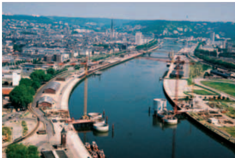
Photo 10 Vue générale socles et gabions General view of bases and gabions
