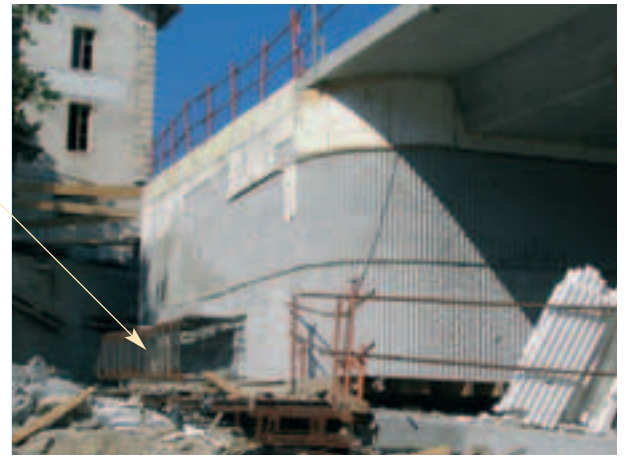
Right bank abutment. Movable upper part. a) Formwork and reinforce- ments (May 2004) - b) Formwork removal in September 2004
