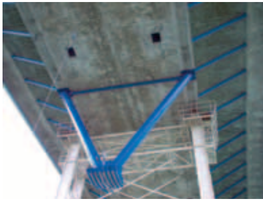
Photo 3 Fixation du poinçon central Fastening the centre truss post
