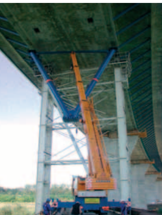
Photo 10 Montage poinçon central Erecting the centre truss post
