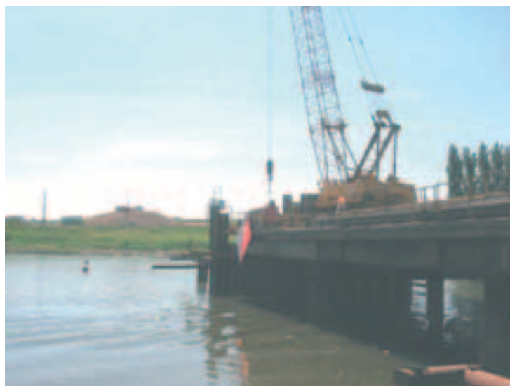
Photo 2 Estacade rive droite Breakwater on the right bank
