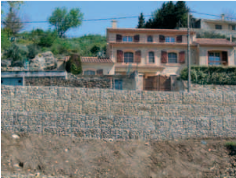
Vue d'ensemble de l'ouvrage fini Overall view of the finished structure
