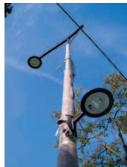
Photo 11 Poteau éclairage et porte-lac Light post and overhead contact line carrier
