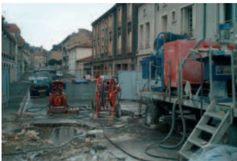
Photo 10 Injections du puits "Sarrail" "Sarrail" shaft cement grouting
