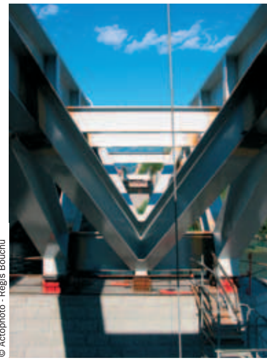
Photo 8 Vue du bracon View of the bracket
