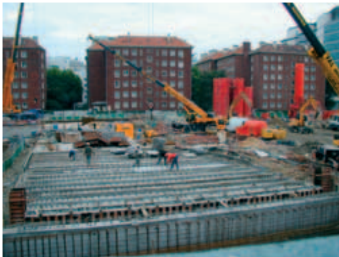
Photo 3 Construction de la dalle supérieure Construction of the upper slab
