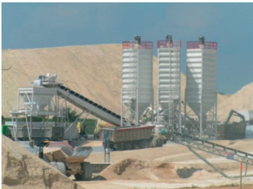
Photo 10 Centrale de Nonant-le-Pin Nonant-le-Pin power station
