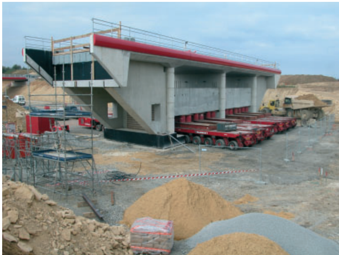
Photo 16 Pont-rail PRA 1309 PRA 1309 railway bridge
