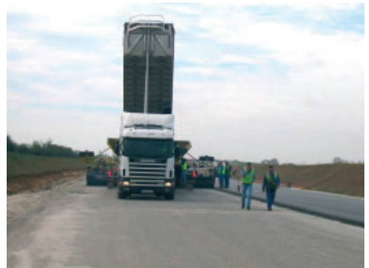
Photo 19 Mise en œuvre grave-bitume Application of bitumen treated base material
