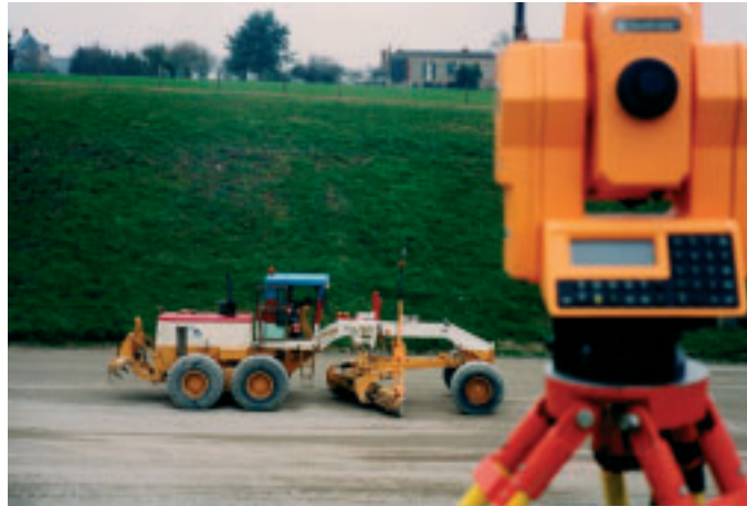
Photo 13 Niveleuse asservie Servo controlled grader
