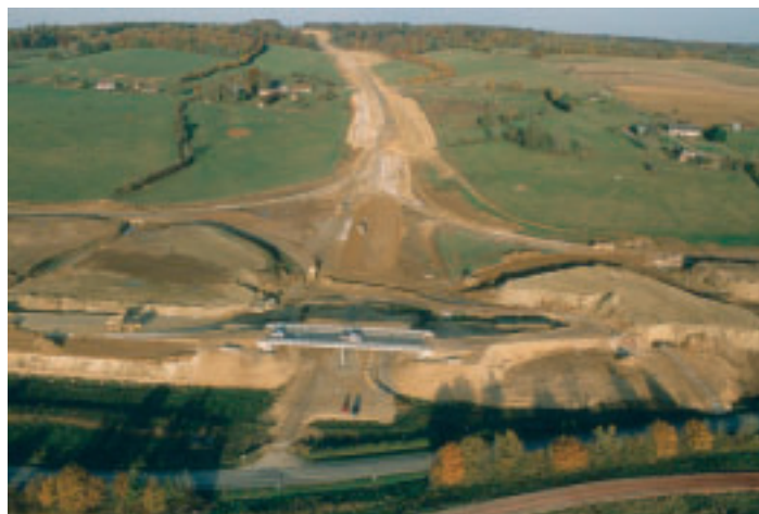
Photo 5 Obstacles Gacé Gacé barriers
