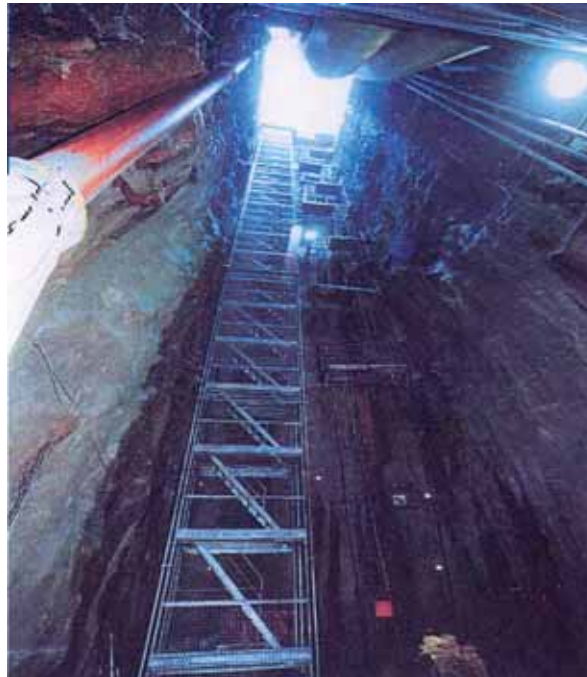
Photo 11 Puits excavé de Kwai Chung Excavated Kwai Chung shaft
