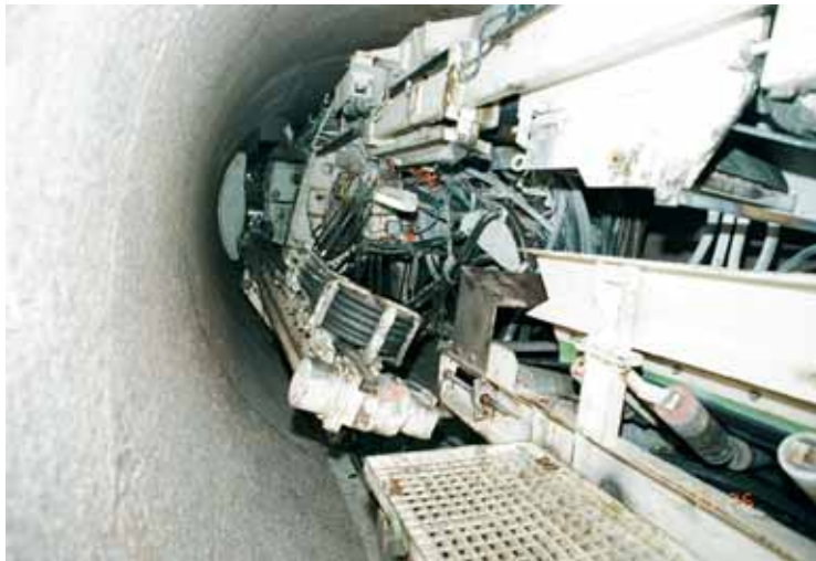
Photo 4 Tunnelier de Chi Ma Wan Chi Ma Wan tunnel boring machine
