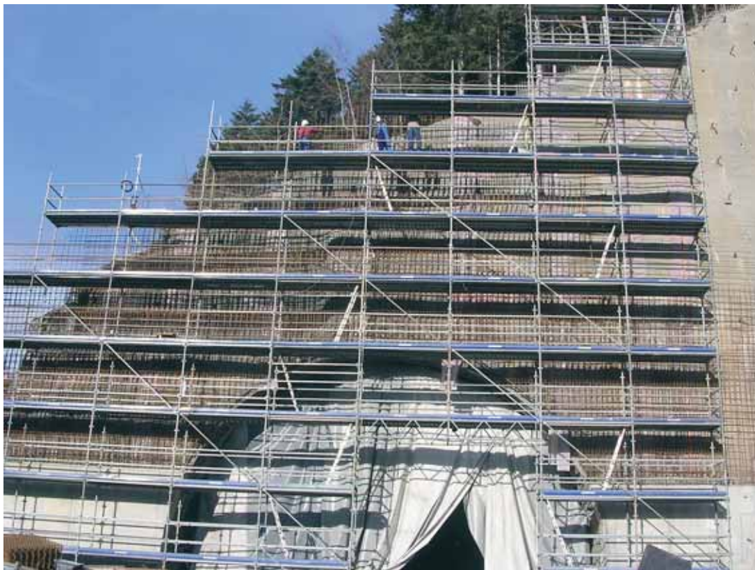
Photo 11 Ferrailage tympan sud-ouest Reinforcement of southwest spandrel
