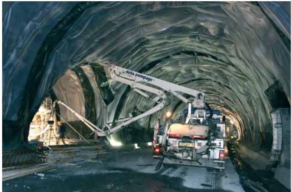
Photo 7 Etanchéité à l'intersection tunnel/by-pass Waterproofing at the tunnel/by-pass intersection
