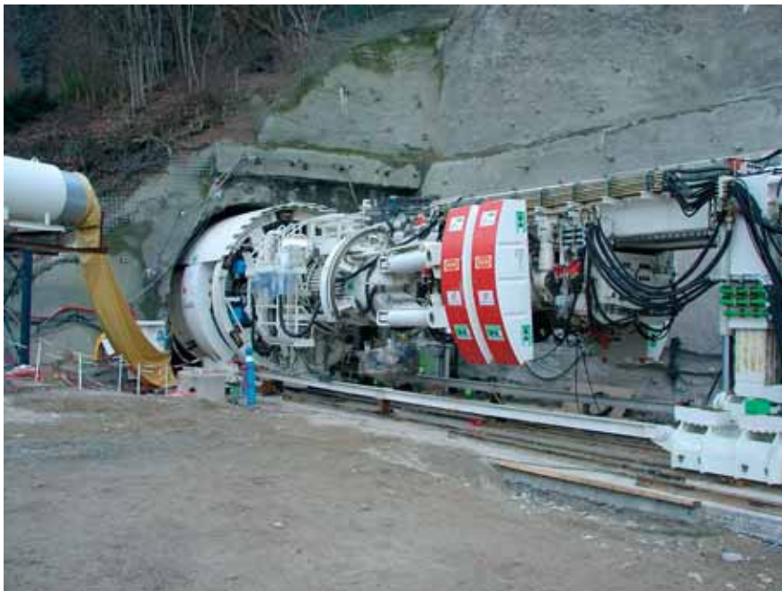
Vue du tunnelier View of the tunnel boring machine
