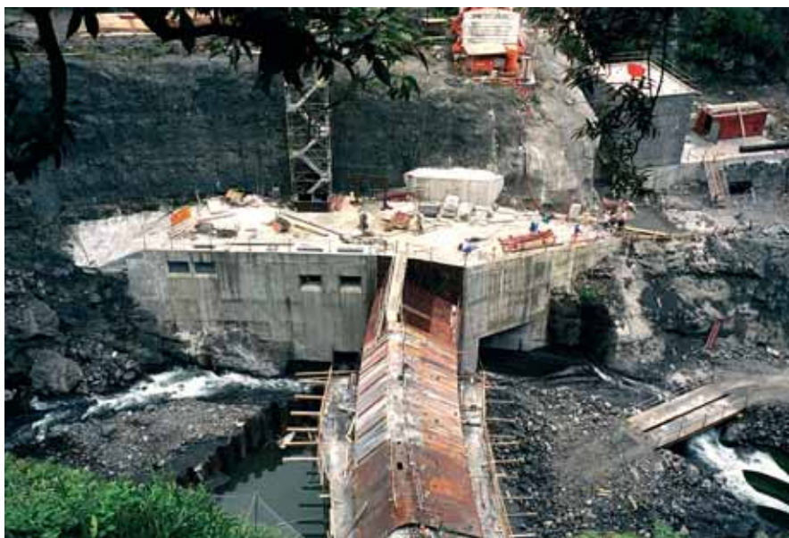
Setting up protective sheets on a weir
