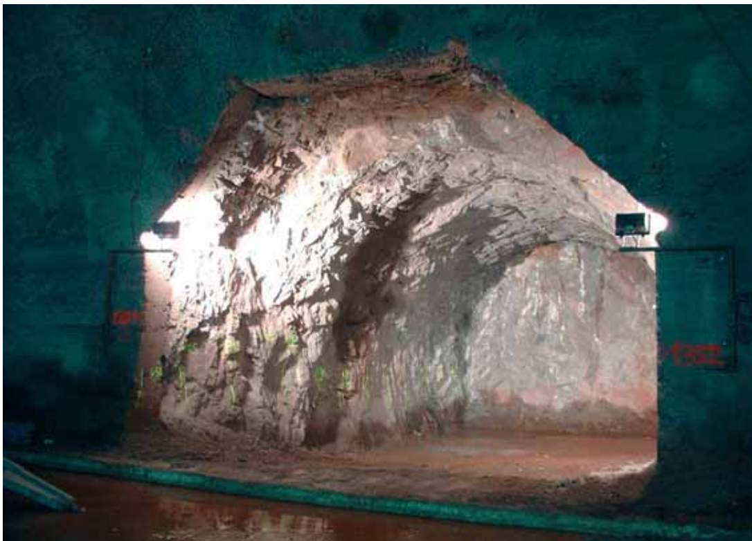
Front tunnel salle de transit Transit room tunnel face
