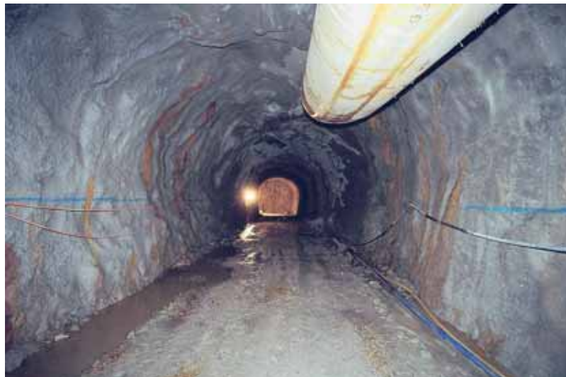
Photo 12 Tunnel excavé de Kwai Chung Excavated Kwai Chung tunnel
