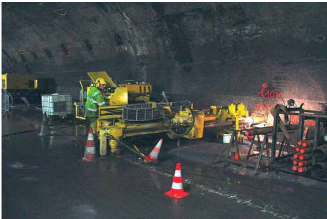
Forage conduits air frais (Mustang) Drilling fresh air ducts (Mustang)
