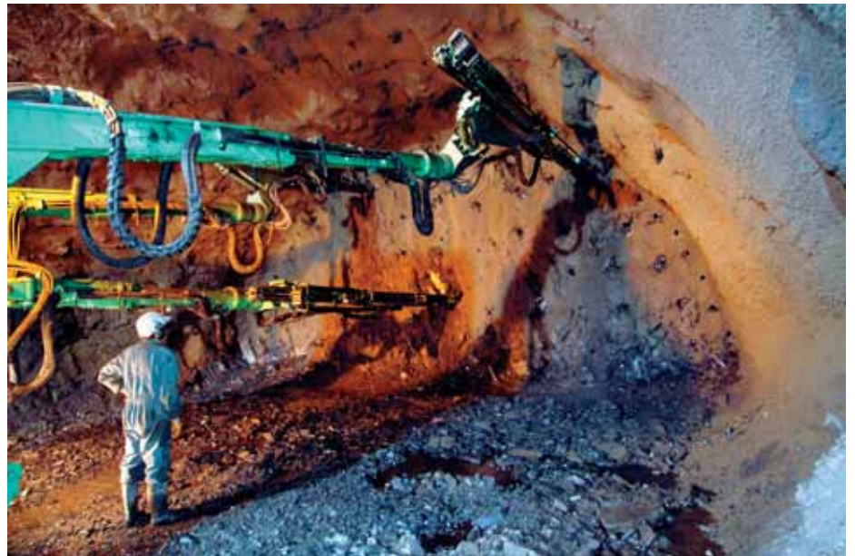
Photo 4 Robofore en foration Robofore during boring
