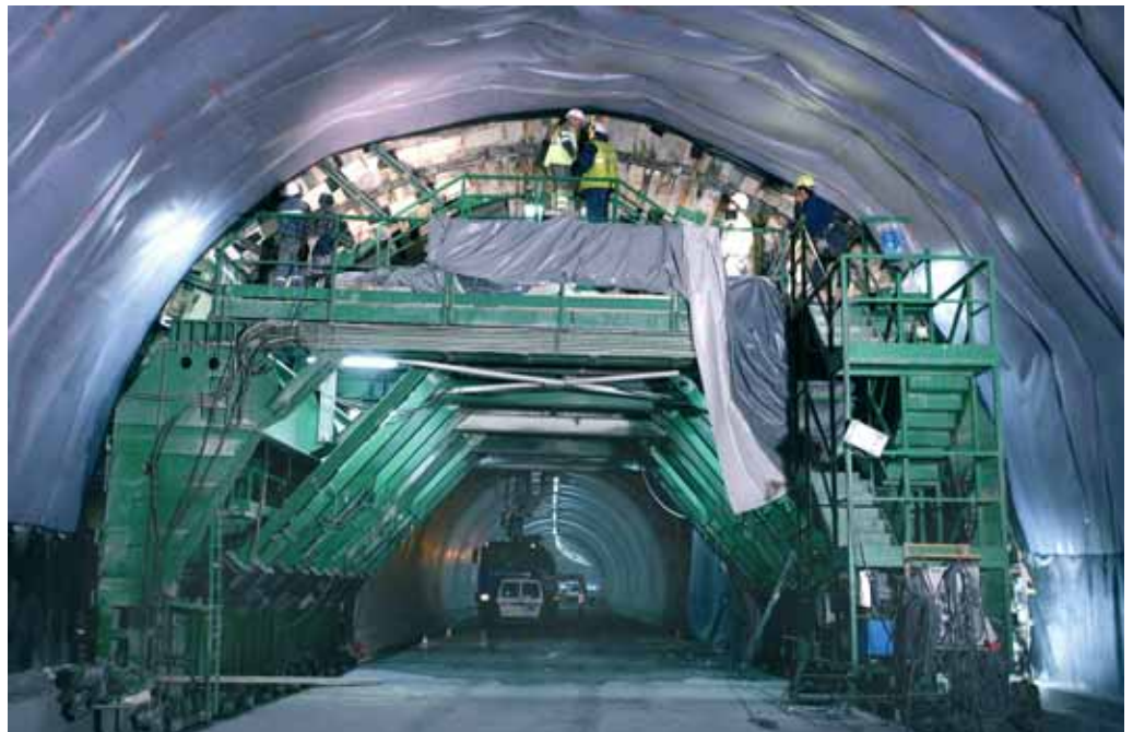
Photo 8 Coffrage en tunnel Shuttering in the tunnel
