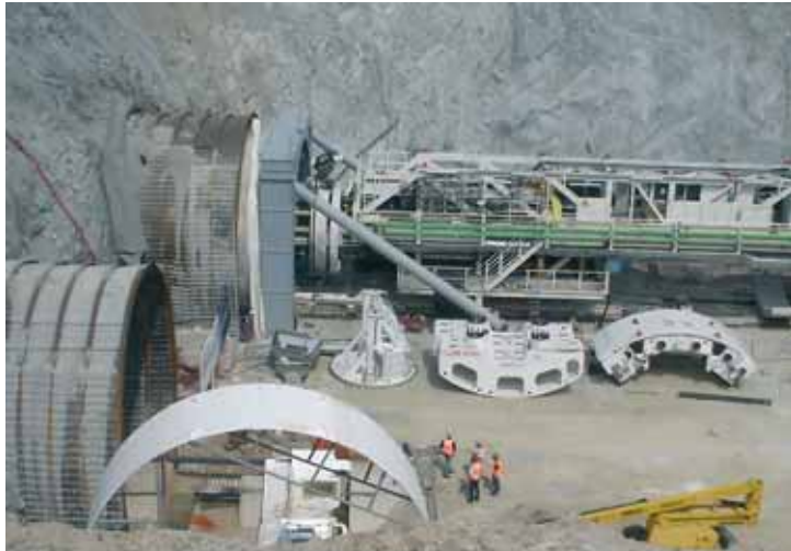
Photo 3 Tunnelier + structure TBM + structure
