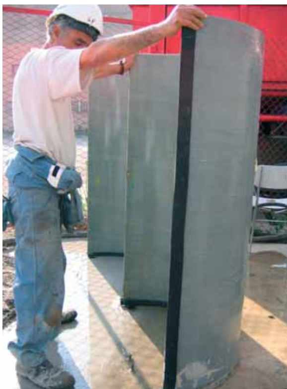
Photo 4 Pose des coques munies de leurs joints d'étanchéité Laying of the shells fitted with their seals
