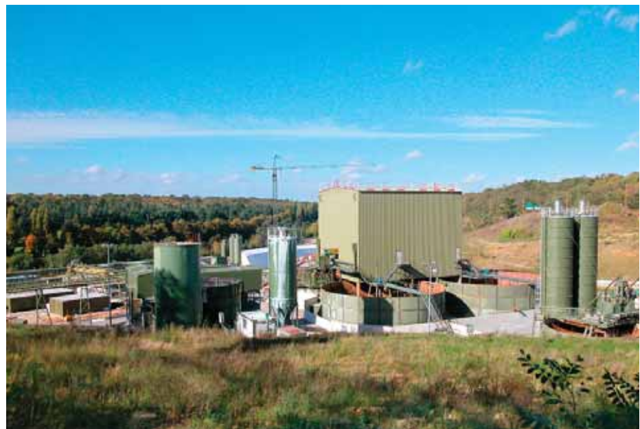
Photo 5 Installations de chantier de Pont Colbert Colbert Bridge construction plant
