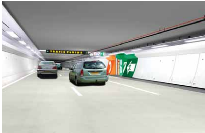
Figure 2 Illustration de l'aménagement intérieur du tunnel Illustration of the interior fittings of the tunnel
