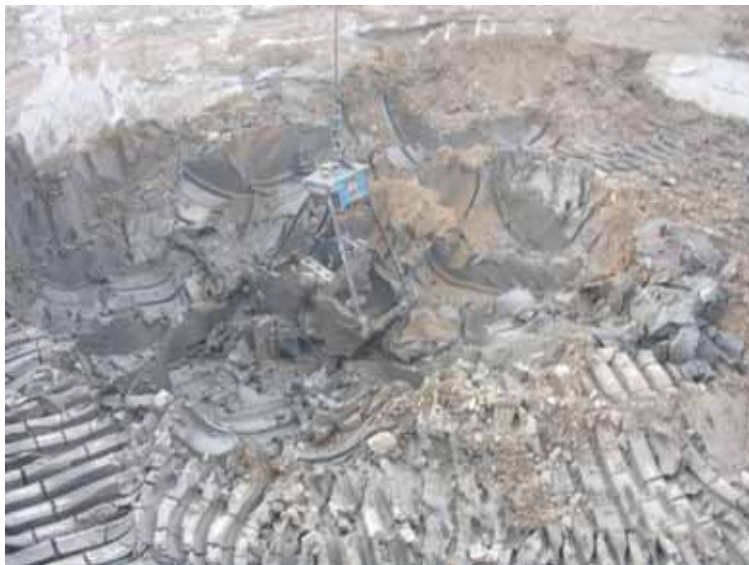
Photo 6 Terrassement P3 Earthworks P3
