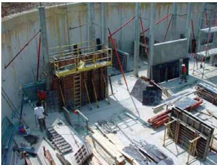
Photo 4 Construction de la structure intérieure Construction of the interior structure
