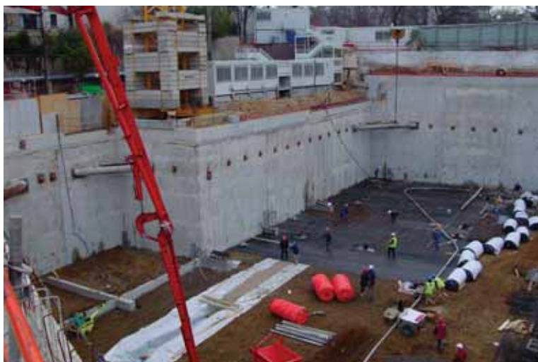
Aperçu de la paroi General view of the wall
