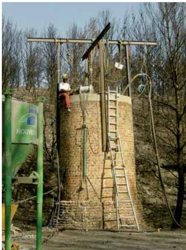
Photo 2 Installation en tête de puits Installation at the shaft head
