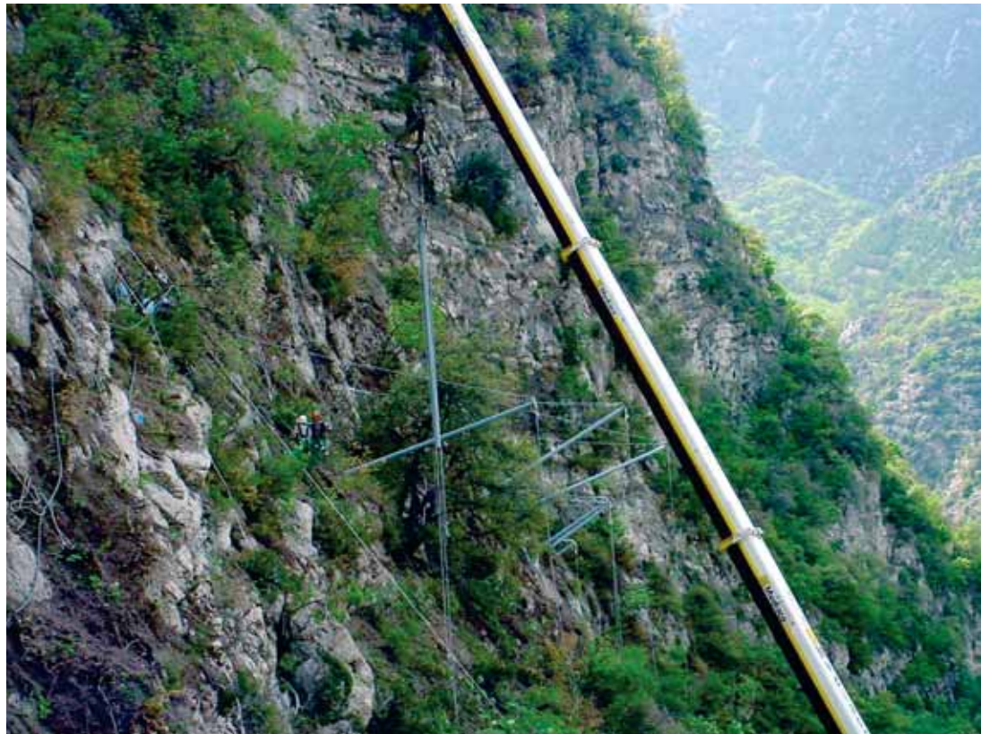
Photo 6 Pose des potences Installing brackets
