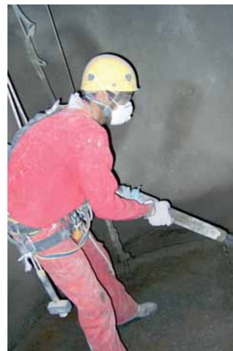
Photo 5 Projection en béton fibré RIG Spraying with "RIG" fibrous concrete
