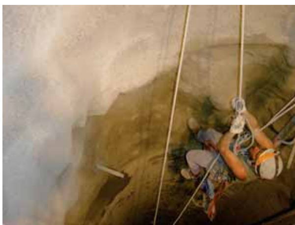
Photo 4 Progression verticale Vertical progress
