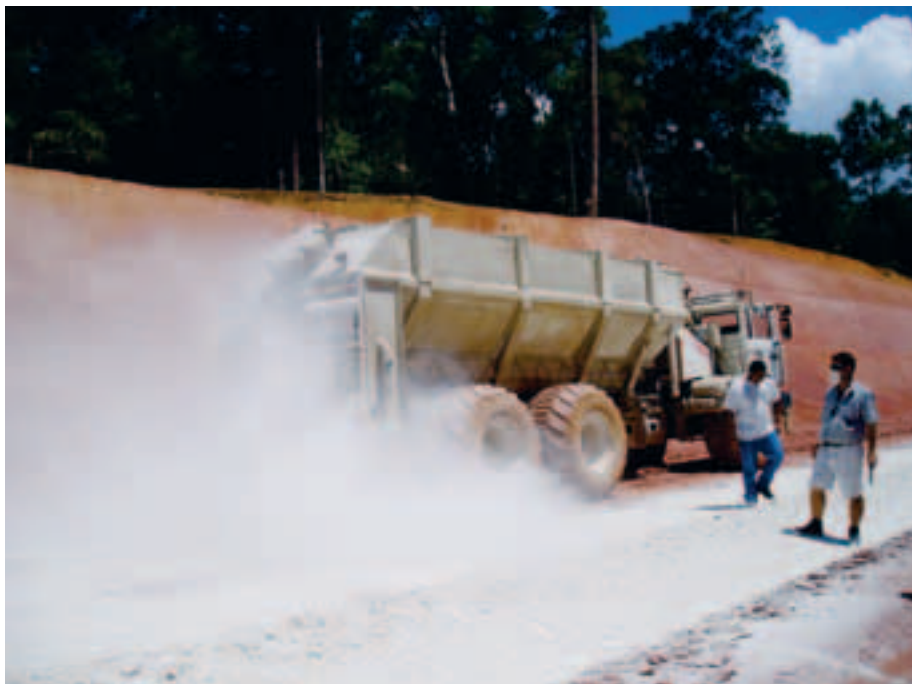
Photo 8 Malaxage en place In-situ mixing
