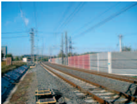
Mur antibruit - Liadur (section Zabori nad Labem - Prelouc)
