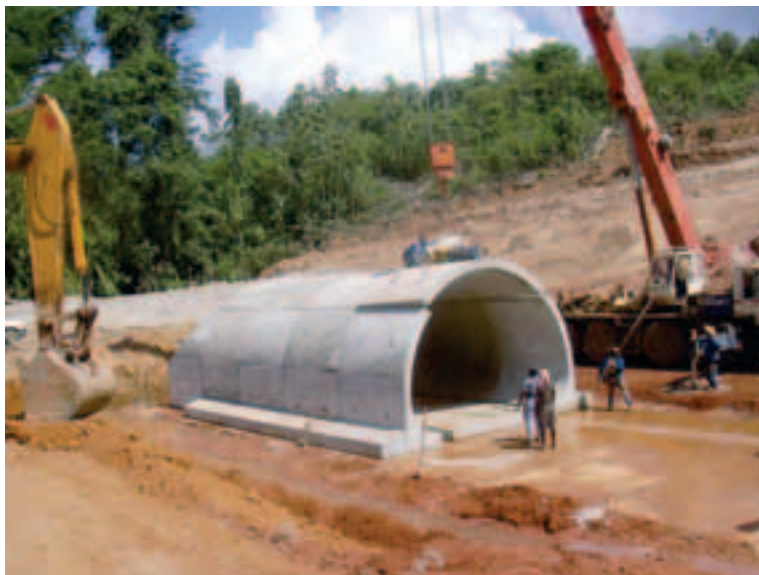
Photo 3 Ouvrage hydraulique Hydraulic structure
