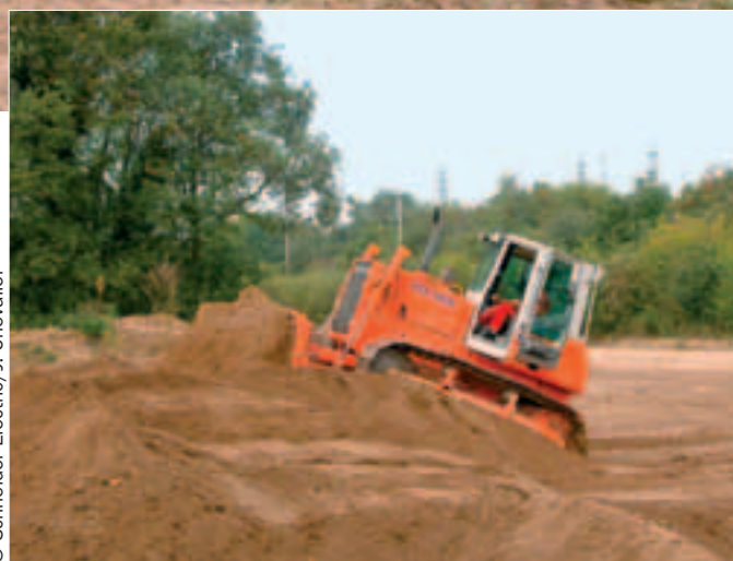
© Schneider Electric/J. Chevallier
