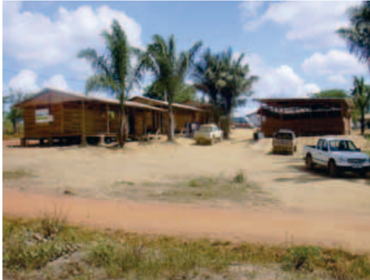
Photo 6 Installation de chantier. Base vie section 6 Site facilities. Construction camp section 6
