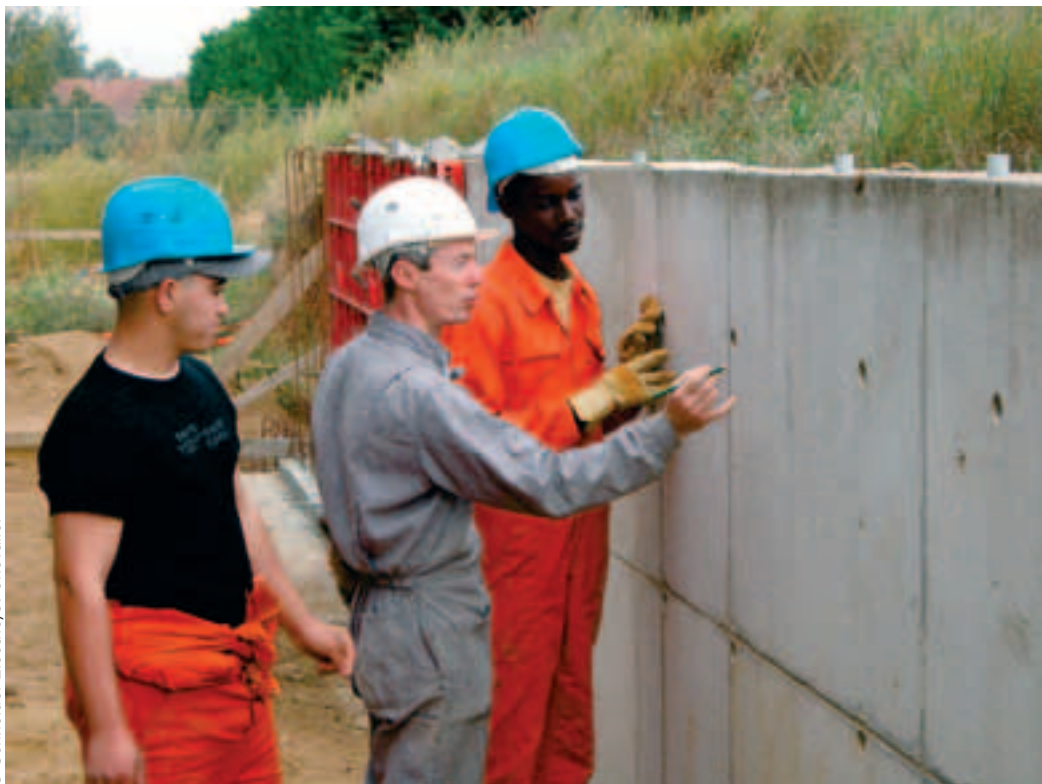
© Schneider Electric/J. Chevallier
