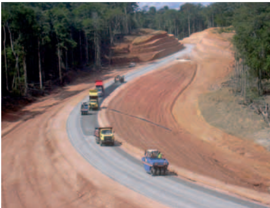
Photo 9 Atelier bi-couche Dual-layer equipment
