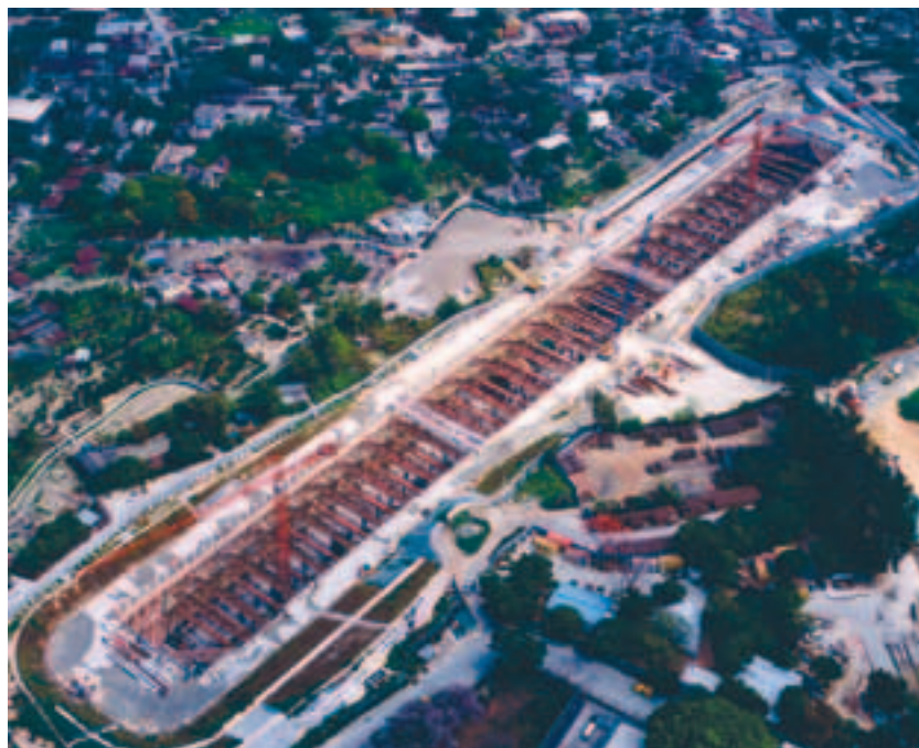
Photo 3 Photo aérienne de la station KTU Aerial photo of KTU station
