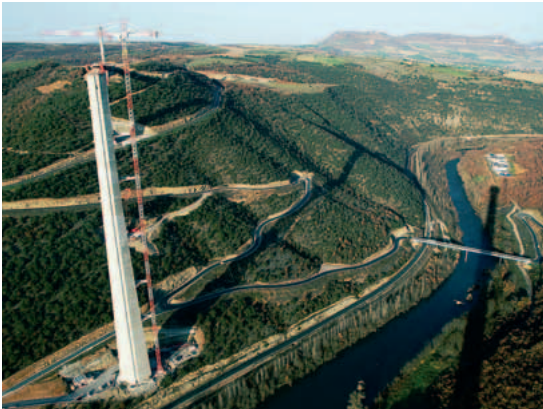
Photo 7 Pile P2. Elévation Pier P2. Elevation view
