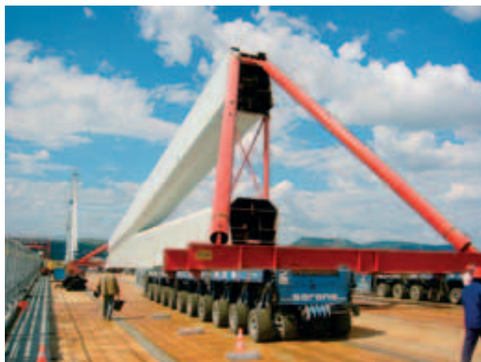
Photo 3 Le transport des pylônes Transporting the towers
