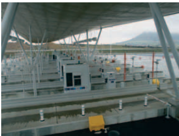
Photo 7 Cabines de péage Toll system booths
