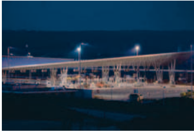
Barrière de péage Toll gate
