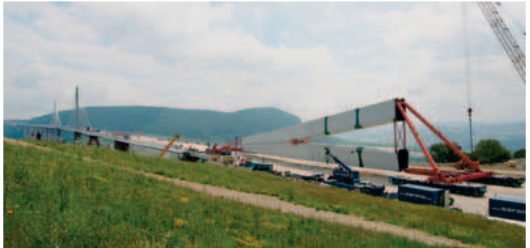
Transport pylône Transporting pylon
