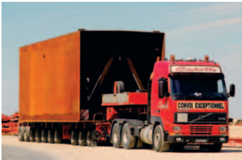
Photo 10 Transport des caissons centraux Transporting the central box girders
