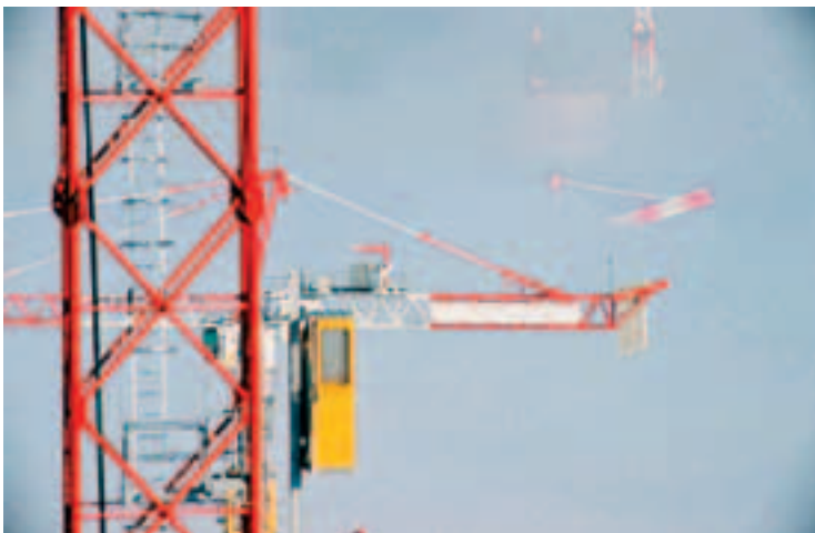
Monte grutier Crane operator lift
