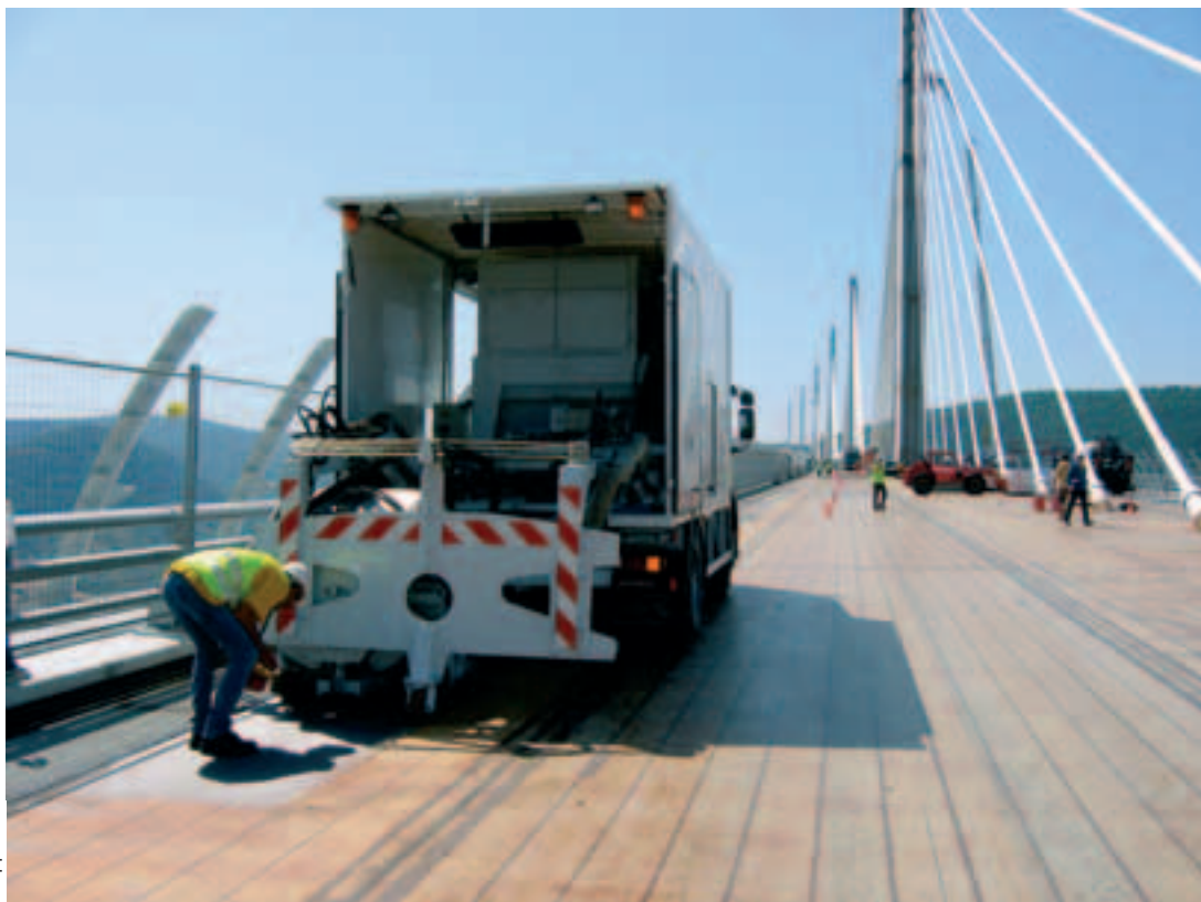
Photo 3 Grenailage Shot blasting
