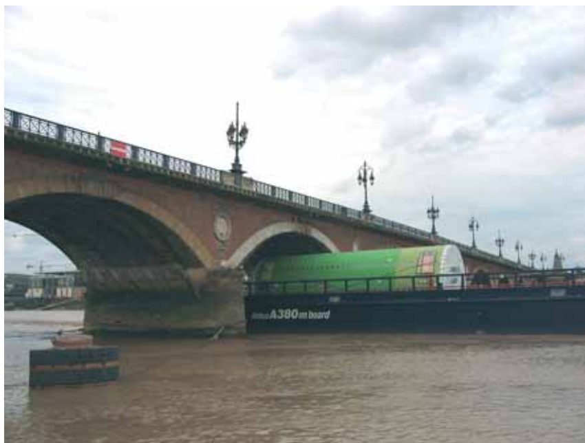
Passage of the Airbus barge under arch No. 11 during work performance
