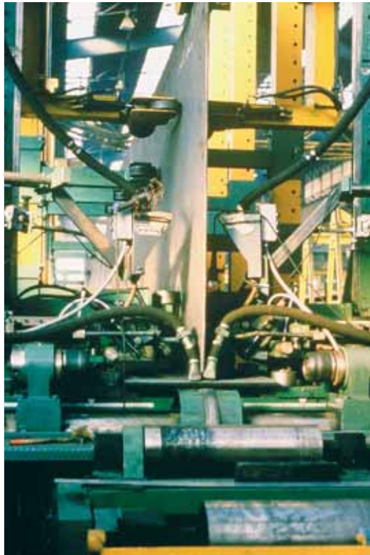
Photo 10 PRS en cours de reconstitution Welded plate girder during welding
