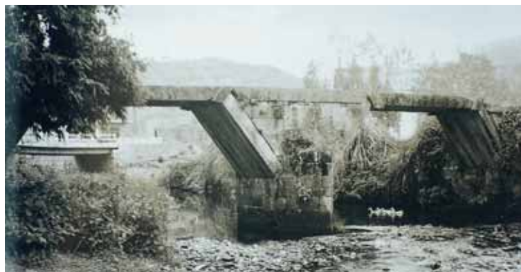
Figure 18a Meixi 3-Fold Arch Bridge. Full view
