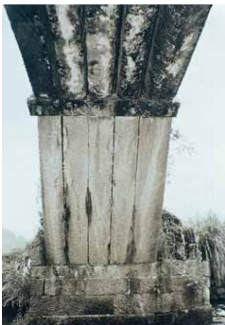
Figure 18b Meixi 3-Fold Arch Bridge. Arch beam
