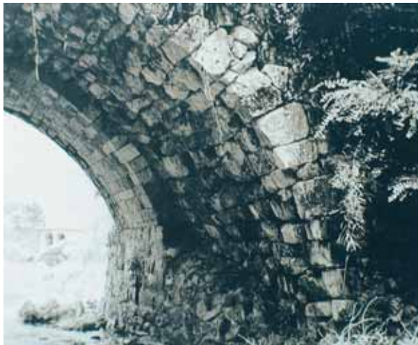
Figure 16 New and old arches of Paishan Bridge
