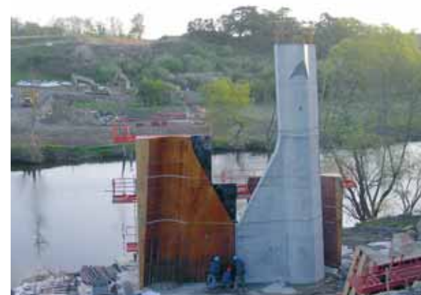
Photo 4 Coffrage bois par demi-pile Wooden formwork for each half-pier
