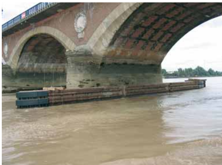
General view of the installed girder
