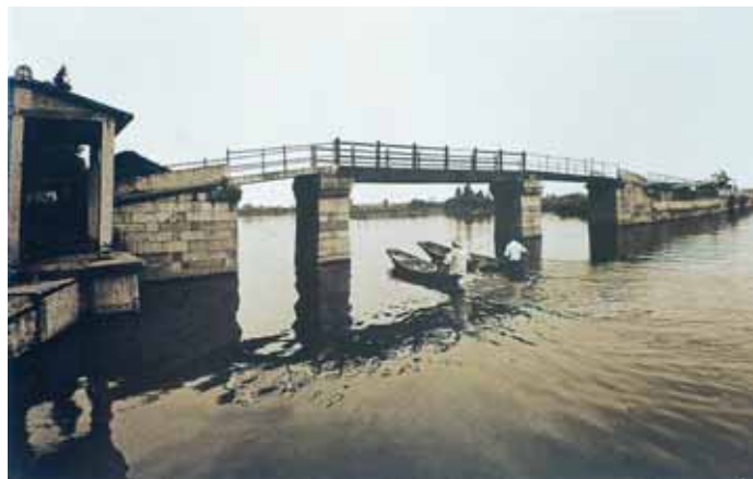
Figure 8 Wanshou Bridge combined with beam bridges and bank
