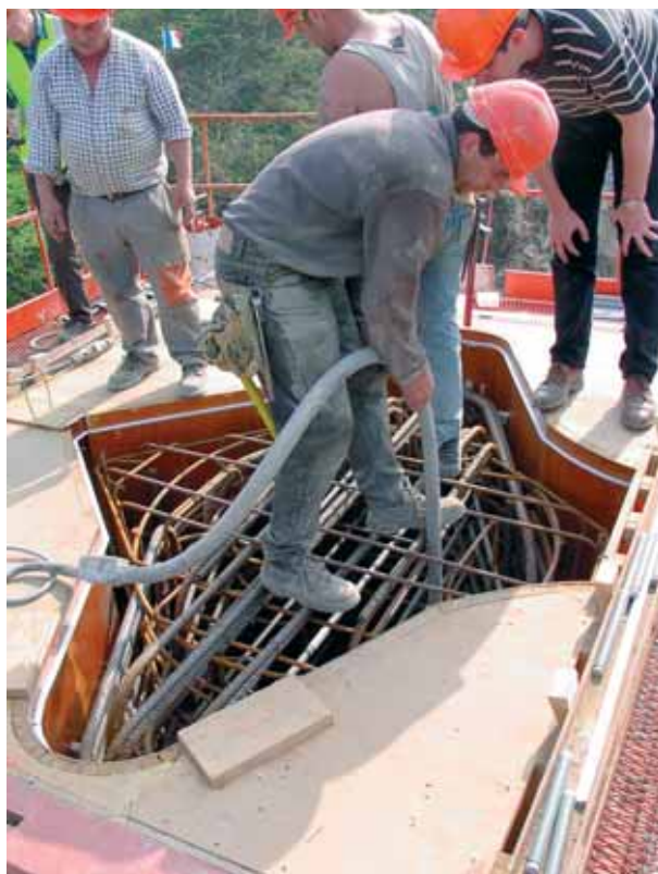
Photo 5 Ferrailage de tête de pile Reinforcement of the pier head
