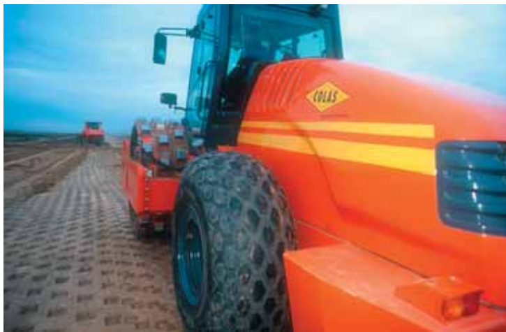
Photo 4 Cylindre vibrant "pied de mouton" "Sheepsfoot" vibratory roller
