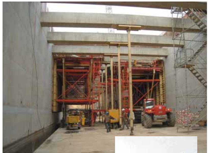
Photo 4 L'outil coffrant en place The sectional formwork in place
