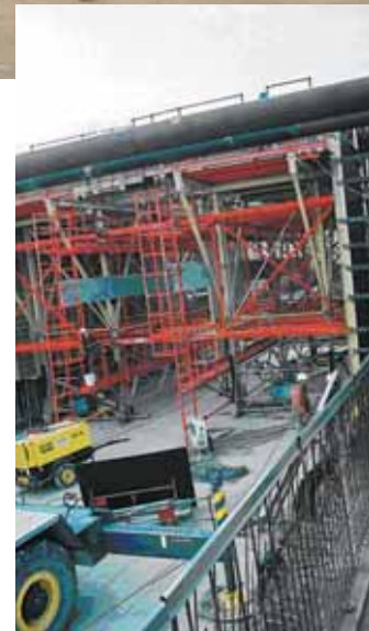
Photo 4 L'outil coffrant en place The sectional formwork in place
