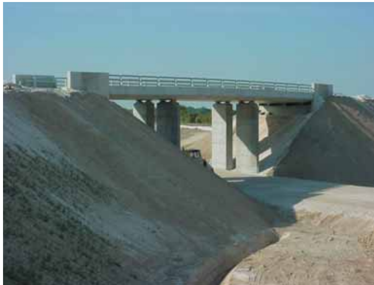
Photo 6 Un pont-route A road bridge
