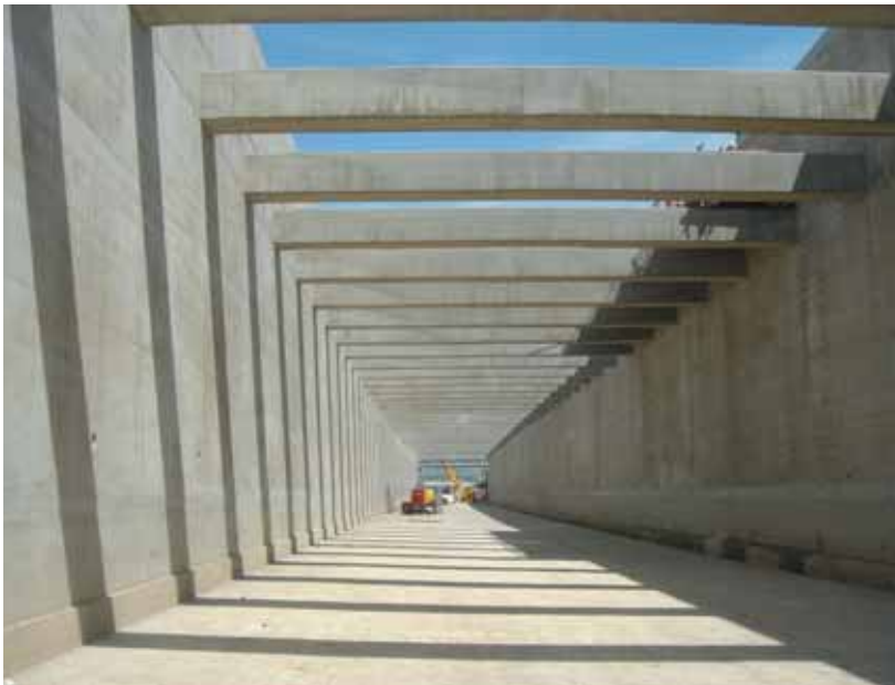
Photo 3 Ouvrage terminé Completed structure
