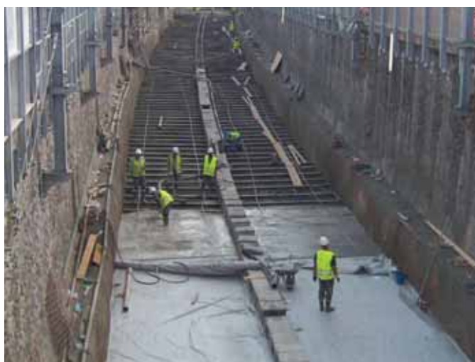
Photo 1 La pose de butons permet la consolidation de l'ouvrage existant Fitting stays to consolidate the existing structure
