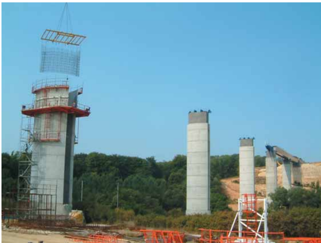
Photo 4 Coffrage grim pant sur pile P5 Climbing formwork on pier P5
