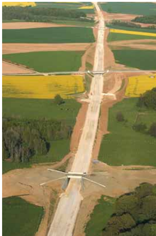
Photo 8 Passage grande faune Underpass for large game
