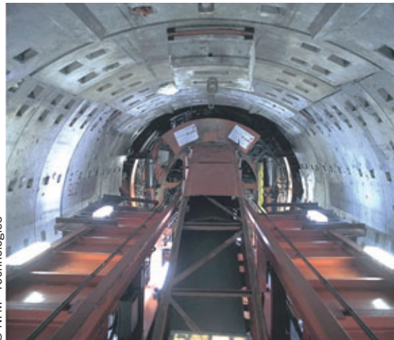
Prefabricated concrete segment, during laying (view of TBM)
