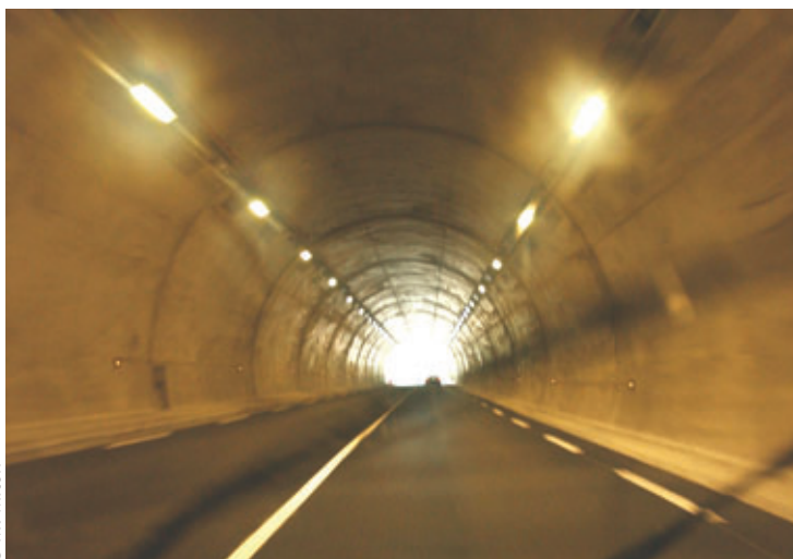
Le tunnel sud The southern tunnel
