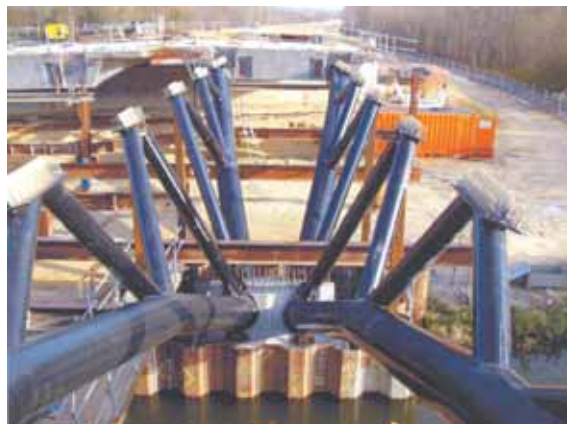
Figure 20 Quatre demi-arcs posés Four half-arches installed
