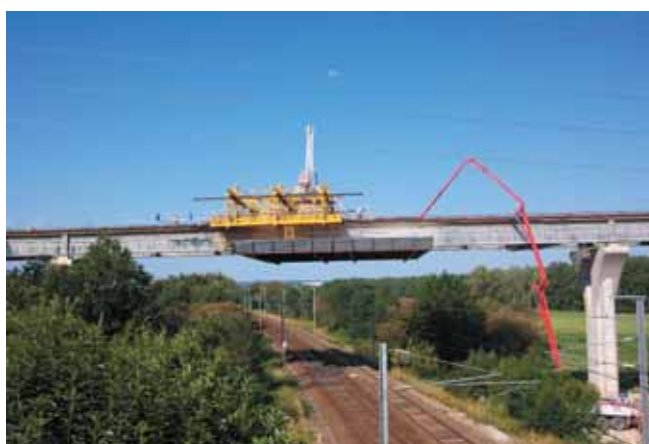
Photo 18 Equipage plot sur voie SNCF Studding rig on railway track
