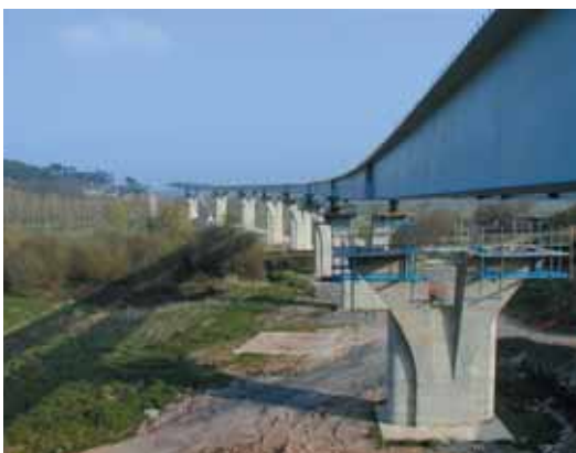
Photo 11 Avancement charpente mars 2002 Structure progress as at March 2002
