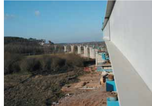
Photo 10 Lancement charpente Structure launching
