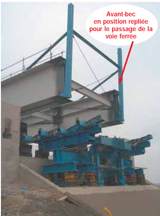
Photo 12 Avant-bec et galets de guidage Launching nose and guide rollers
