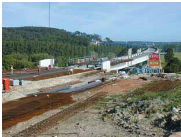
Photo 15 Préfabrication armatures tablier Prefabrication of deck reinforcements
