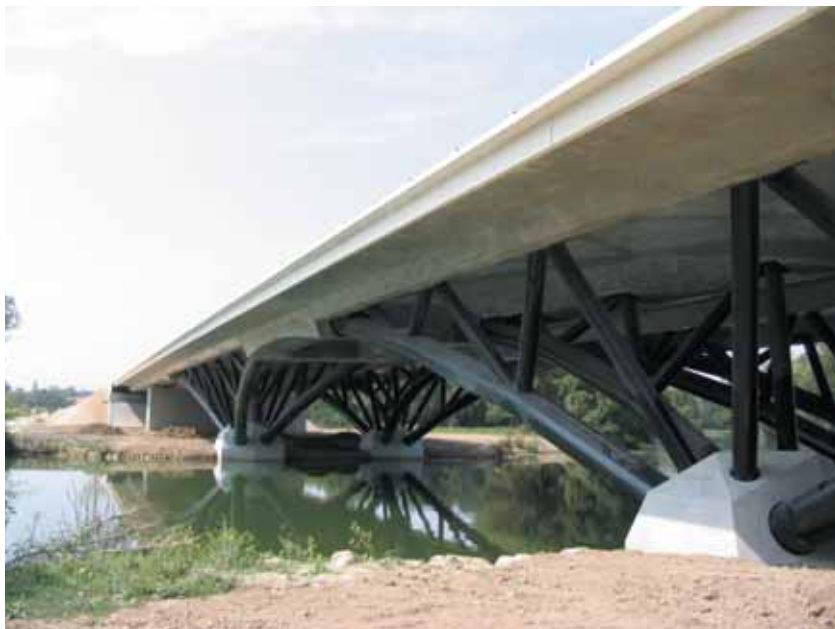
Figure 30 Ouvrage terminé - Ensemble Completed structure - General
