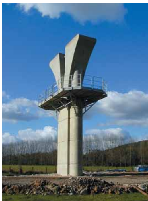
Photo 6 Pile terminée Completed pier
