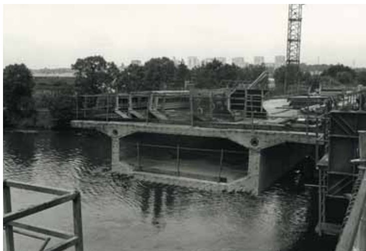
Photo 4 Caisson Box girder
