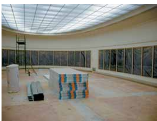
Photo 5 Protection anti-poussière Protection against dust
