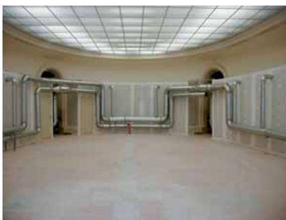
Photo 6 Protection lourde Heavy protection
