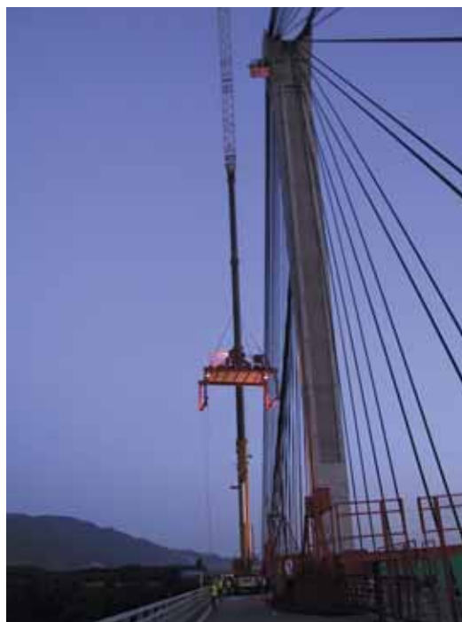
Installation of the tower-head foot bridge. Lifting the podium on the left and one of the two external side foot bridges on the right
