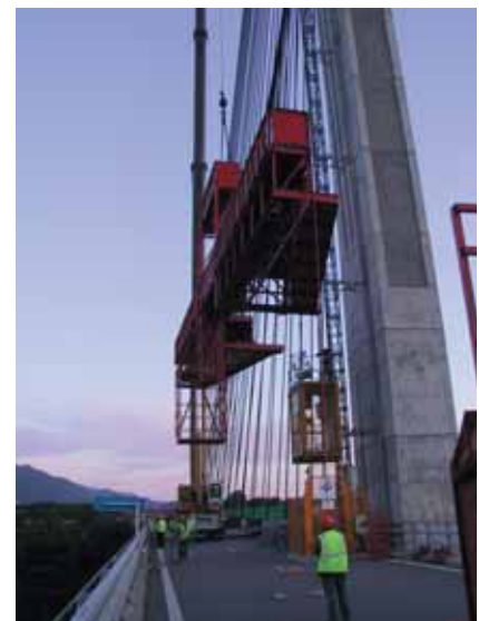
Installation of the tower-head foot bridge. Lifting the podium on the left and one of the two external side foot bridges on the right
