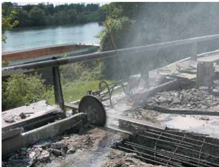
Photo 6 Sciage Sawing
