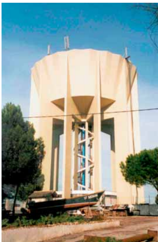
Photo 6 Ravalement terminé Completed resurfacing
