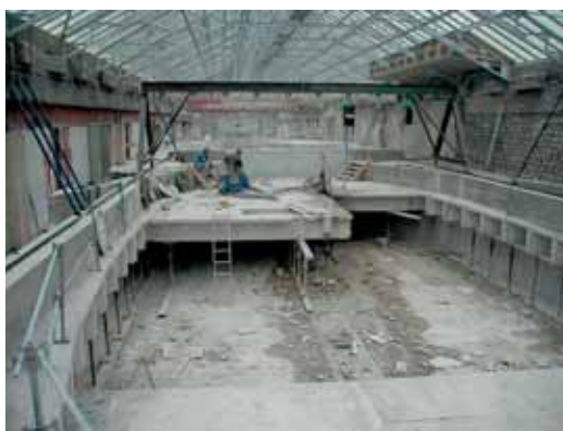
Photo 3 Sciage des planchers Sawing floors
