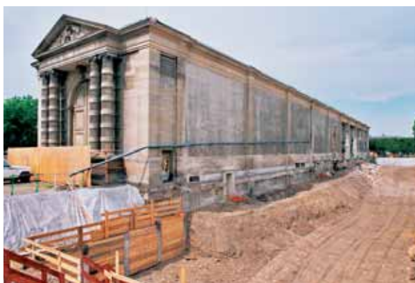
Photo 5 Protection anti-poussière Protection against dust
