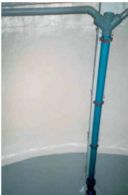
Photo 8 Intérieur fini de la cuve Finished inside of the tank
