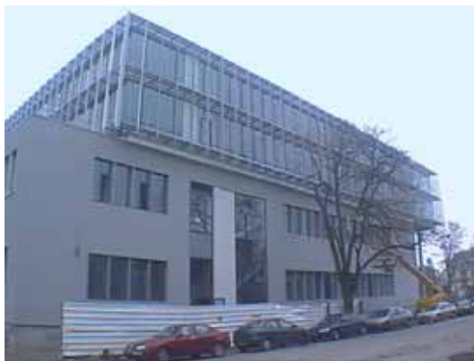
Photo 2 Façade sud du bâtiment South facade of the building
