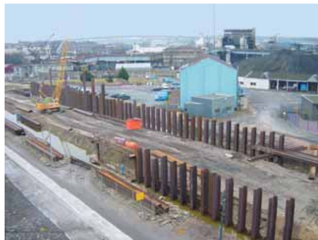
Photo 2 Battage du rideau mixte Pile driving of the combined curtain
