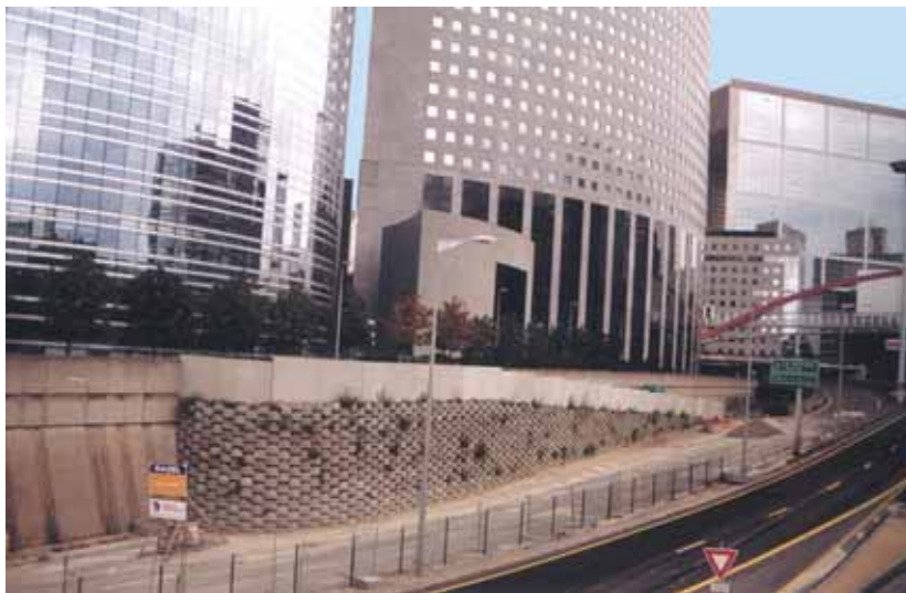
Photo 5 Vue globale de l'ouvrage fini Overall view of the finished structure
