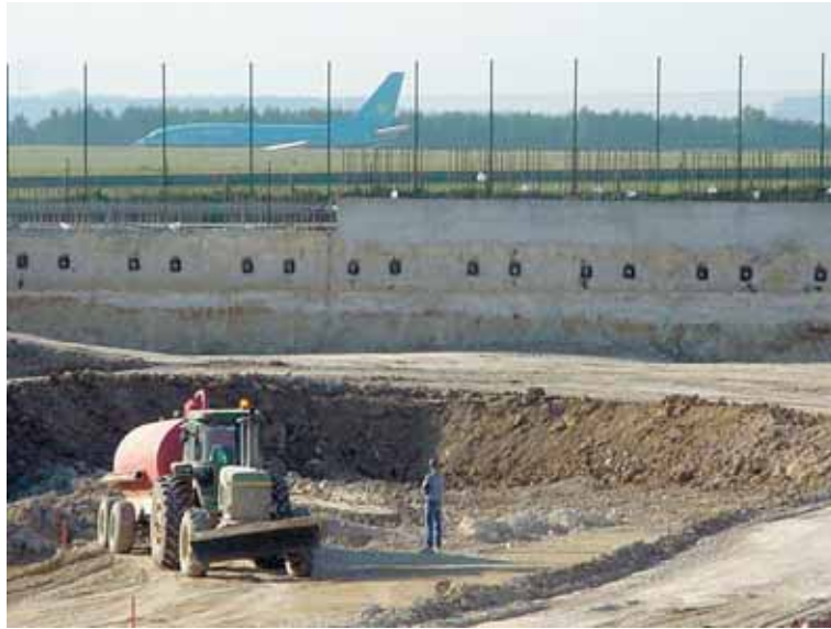
Les tirants provisoires Temporary tension members
