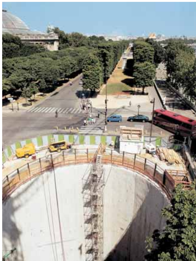
Le puits terminé The completed shaft
