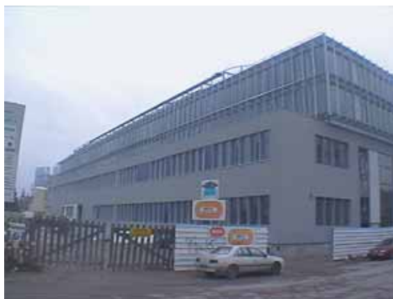
Photo 3 Façade ouest West facade
