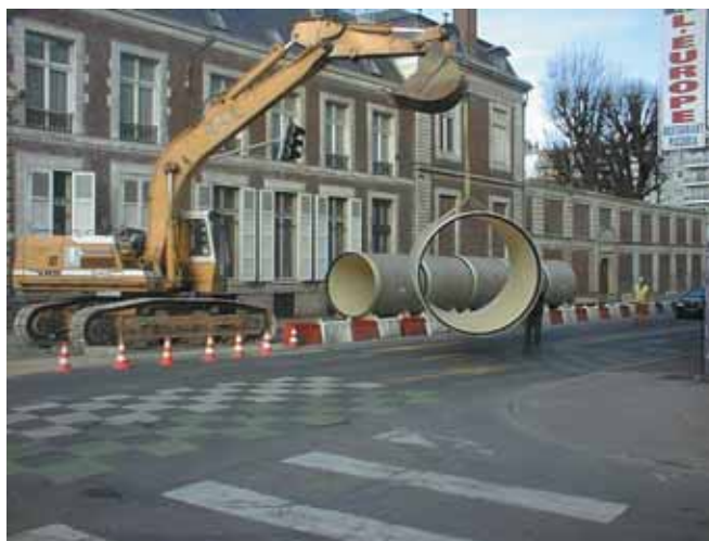
Photo 2 Manipulation d'un tuyau Handling a pipe
