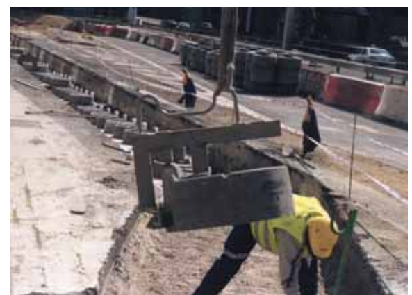
Photo 1 Manutention des cellules béton Handling the concrete cells
