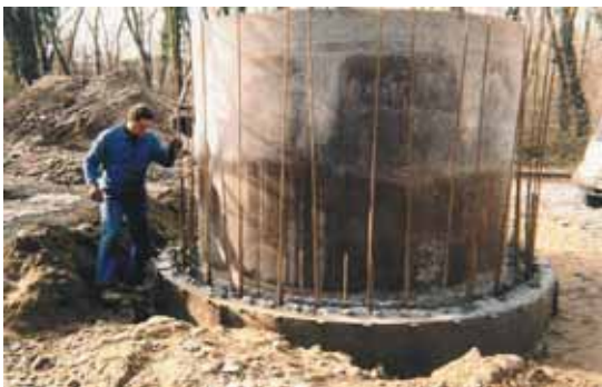
Photo 5 Coffrage et ferrailage Shuttering and reinforcement
