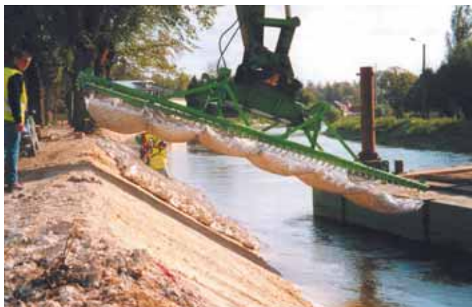
Photo 9 Pose des matelas Mattress laying
