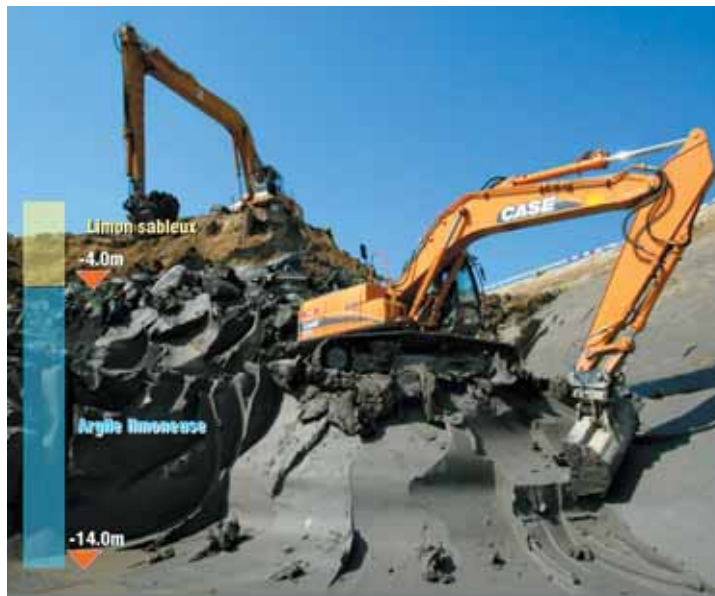
Photo 1 Coupe de terrain Cross section of ground
