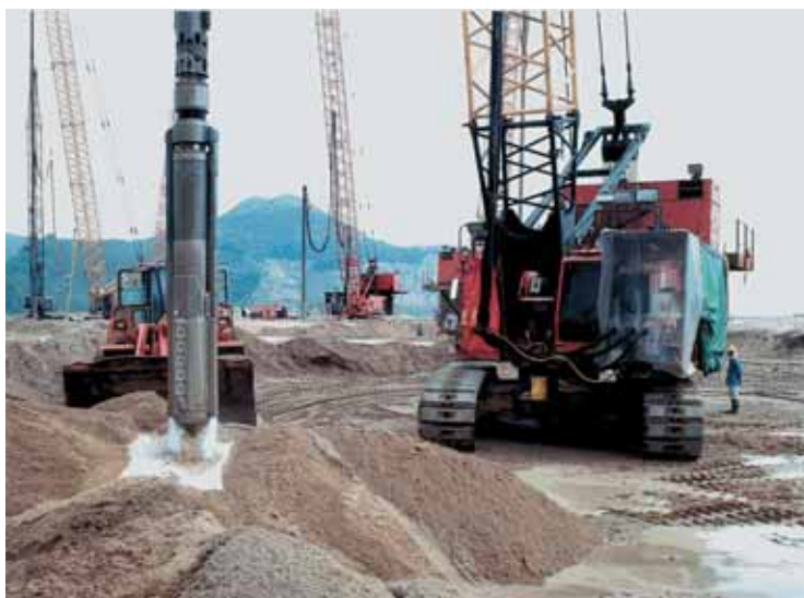
Photo 3 Vibreux en action A vibrator at works
