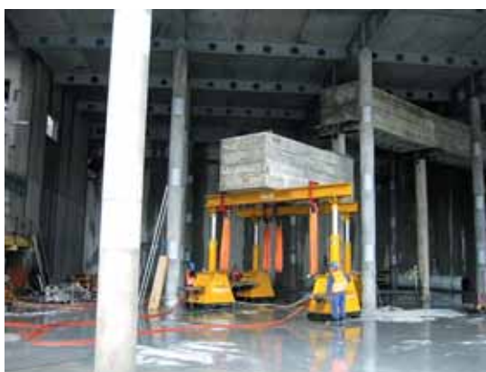
Photo 15 Dépose - Descente éléments Laying down Lowering of elements
