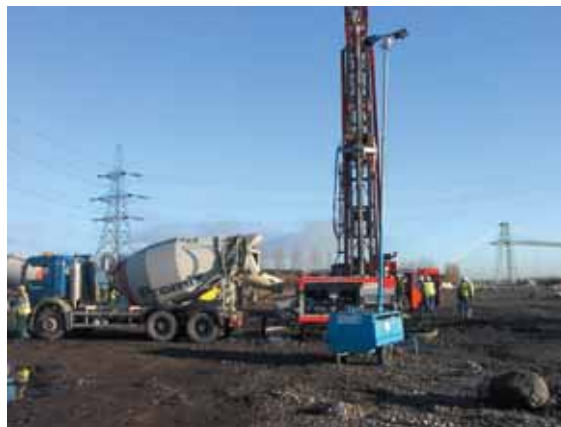
Atelier de CMC et toupie béton CMC equipment and ready mix concrete truck
