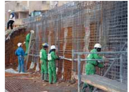
Photo 3 Poste ferrailage profil 2 Reinforcement station profile 2
